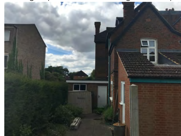
Image 3 (eastern facing elevation and area of flat roof)
