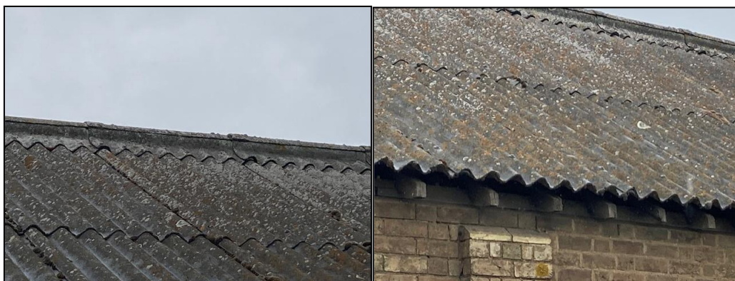
Photographs 5 - 6: Corrugated asbestos roof
