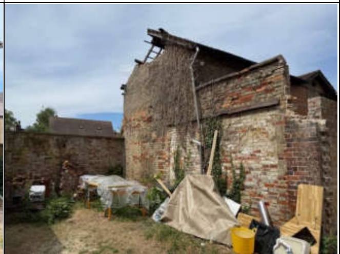
Photo 4 – View of existing structure looking west.
