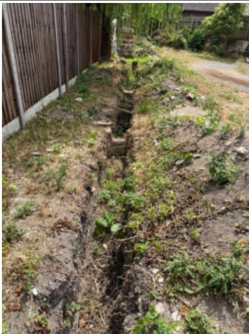
Photo 11 – Exposed trench along the northern site boundary.
