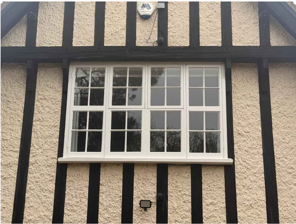
Existing External Window Elevation Image
