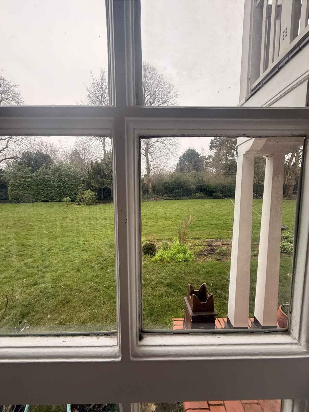
Existing Window Profile Image
