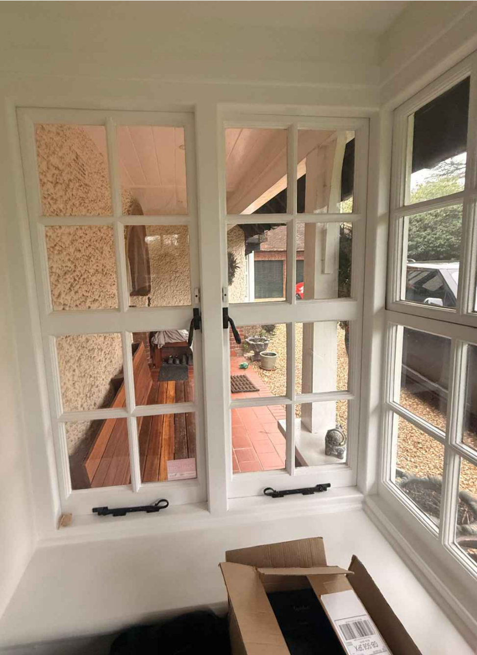
Existing Window Internally Image
