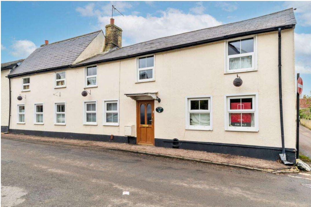
Photo 2 – Front Elevation on Back Street
