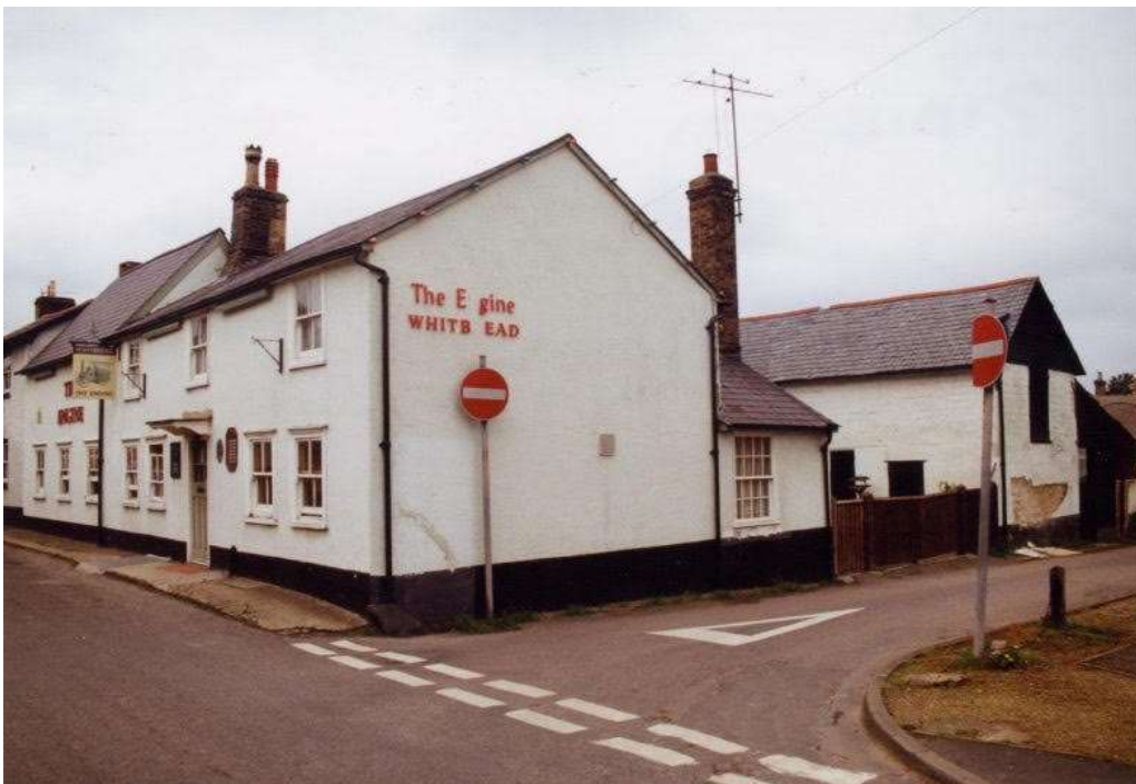
Photo 6 – From 1991 showing a since demolished large barn to the rear
