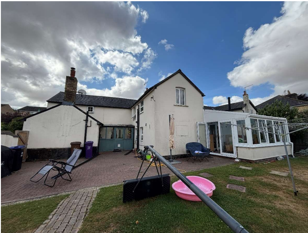
Photo 5 – Rear Elevation showing the current disconnect from the garden to the Library, Kitchen & Dining spaces
