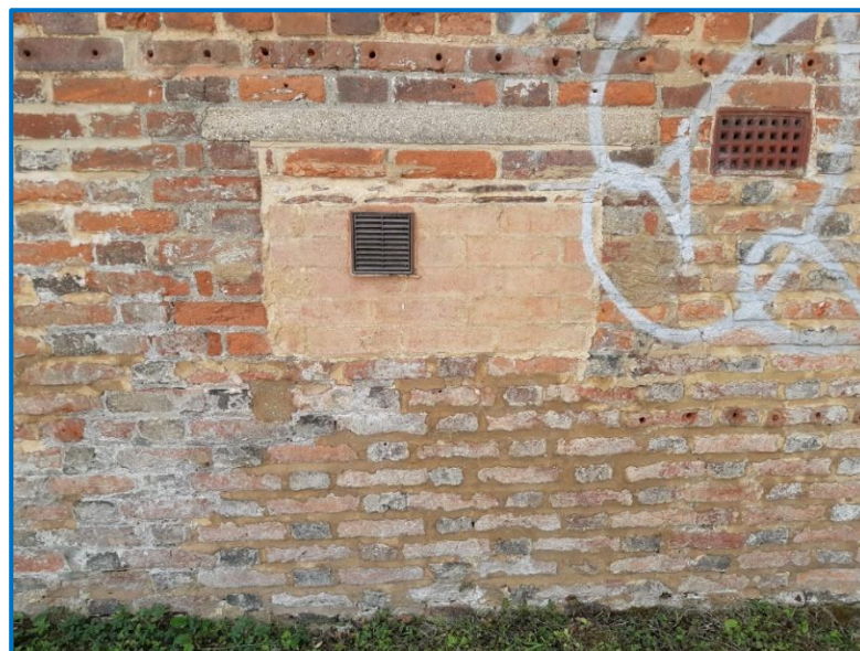
Figure 10 - Bricked up former window and lintel on rear elevation
