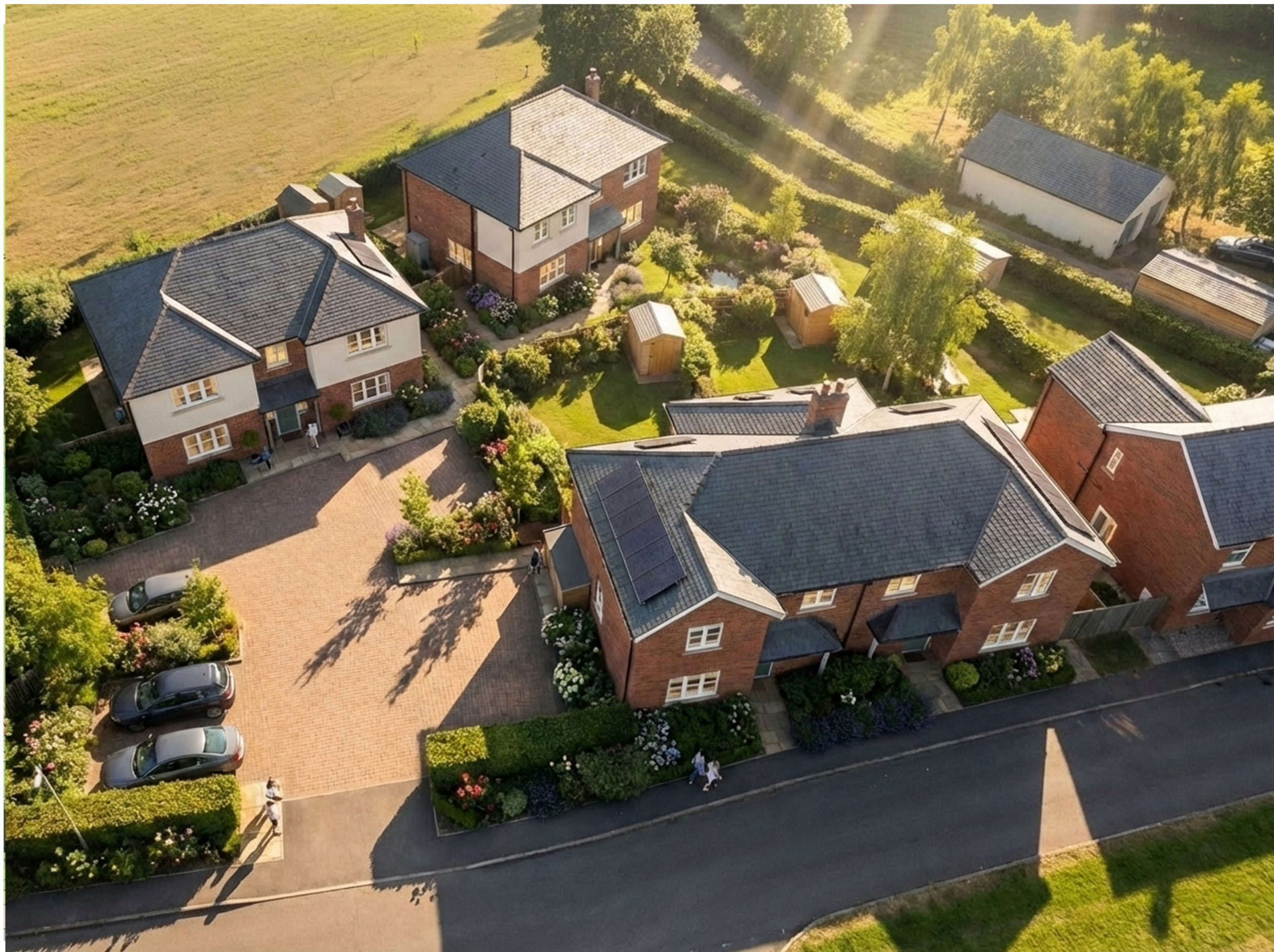
Aerial View from North
