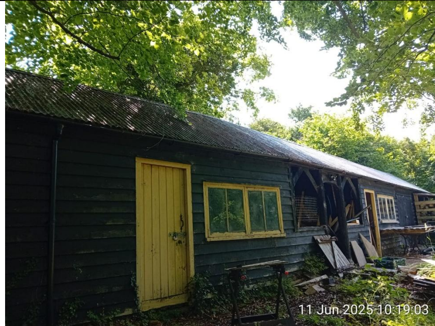
Figure 2: Front elevation of B1
