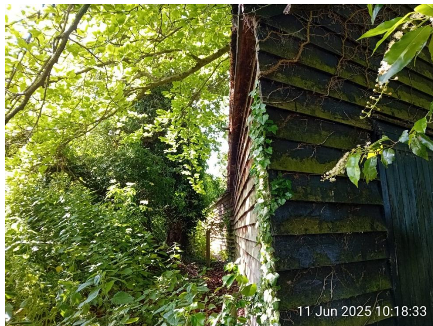
Figure 3: Rear elevation of B1
