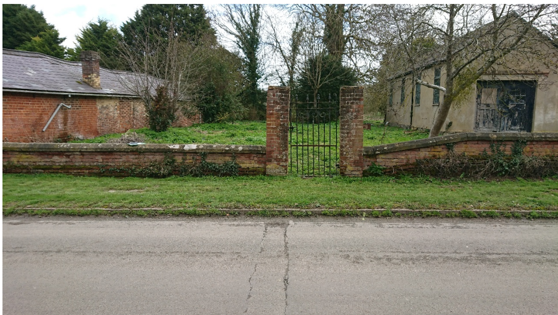
Image showing existing pedestrian access to the Generator Building
