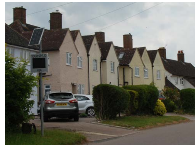
1930's housing along Station Road, north of the application Site
