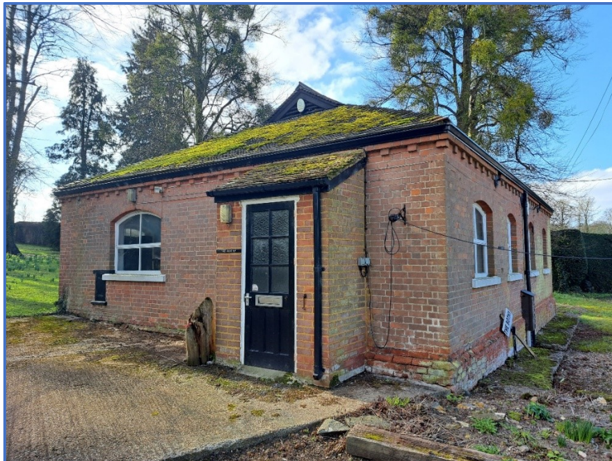
Figure 2 – View of The Bothy – East elevation
