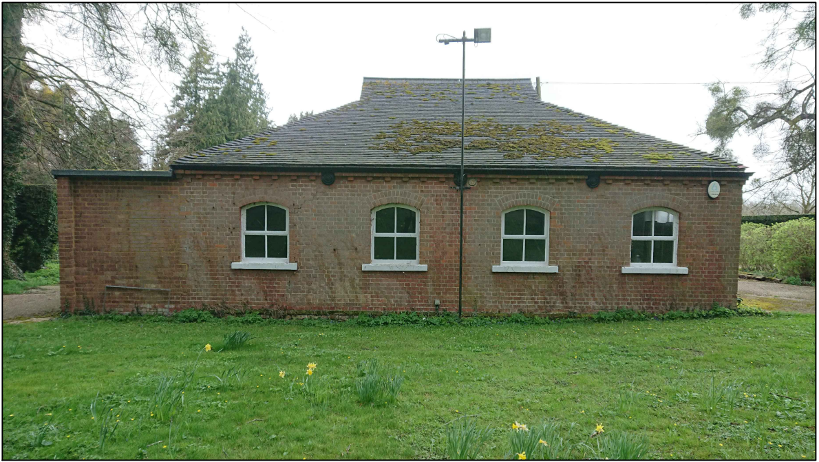
Existing Bothy Image (South)
