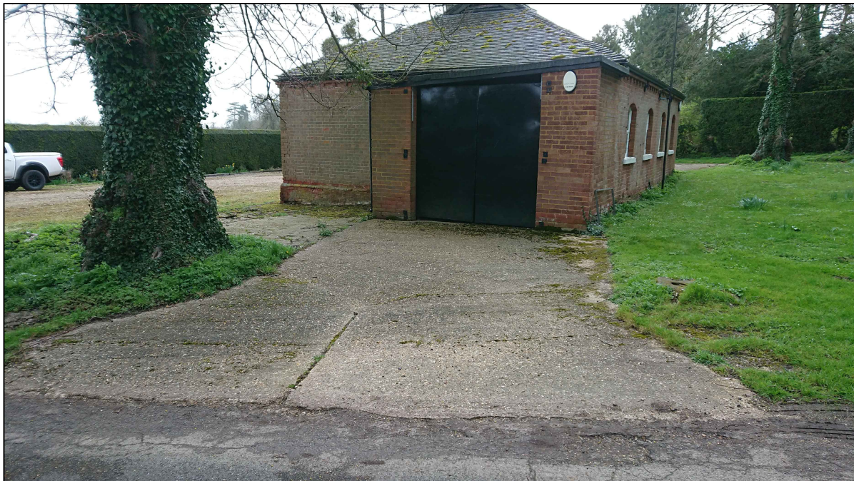
Existing Bothy Image (West)
