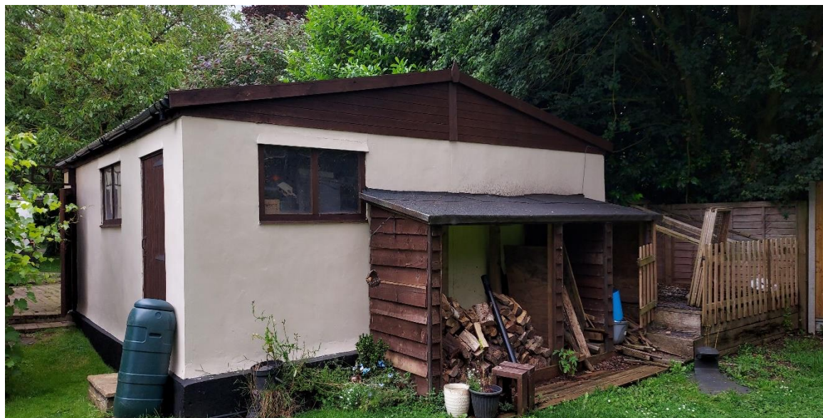
Rear elevation of Garage
