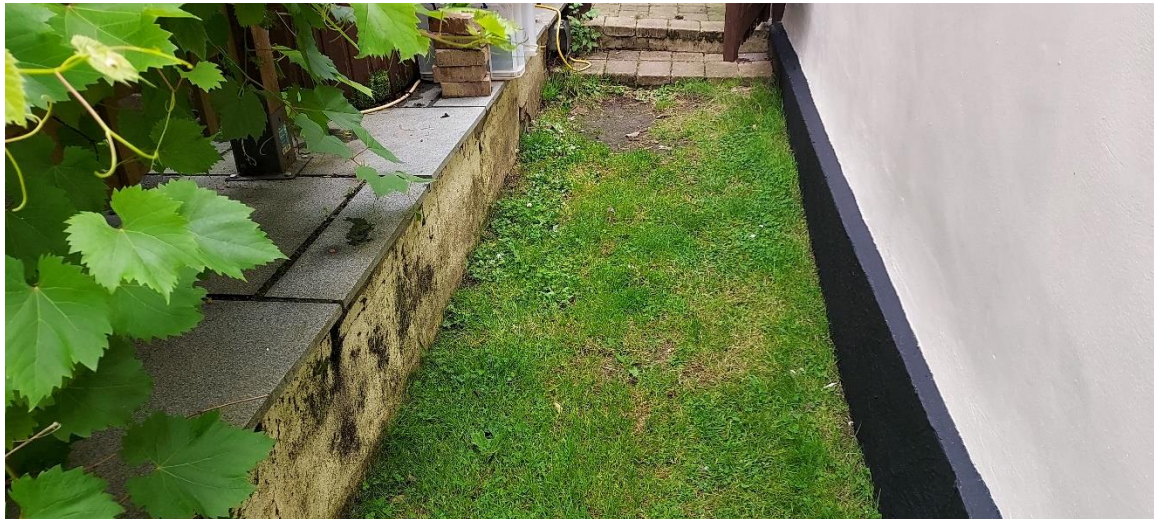
Garage adjacent rear raised patio area
