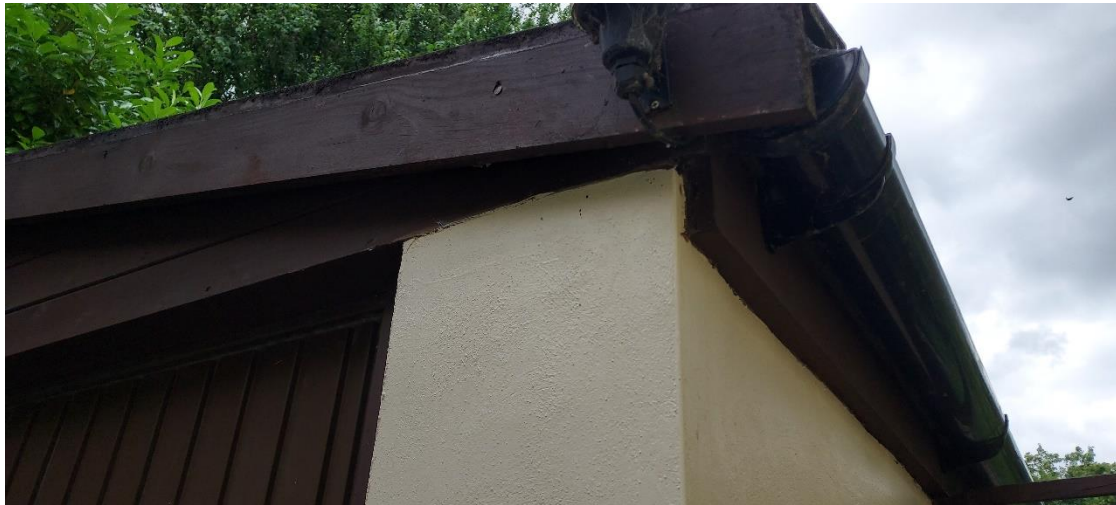
Garage front eaves detail
