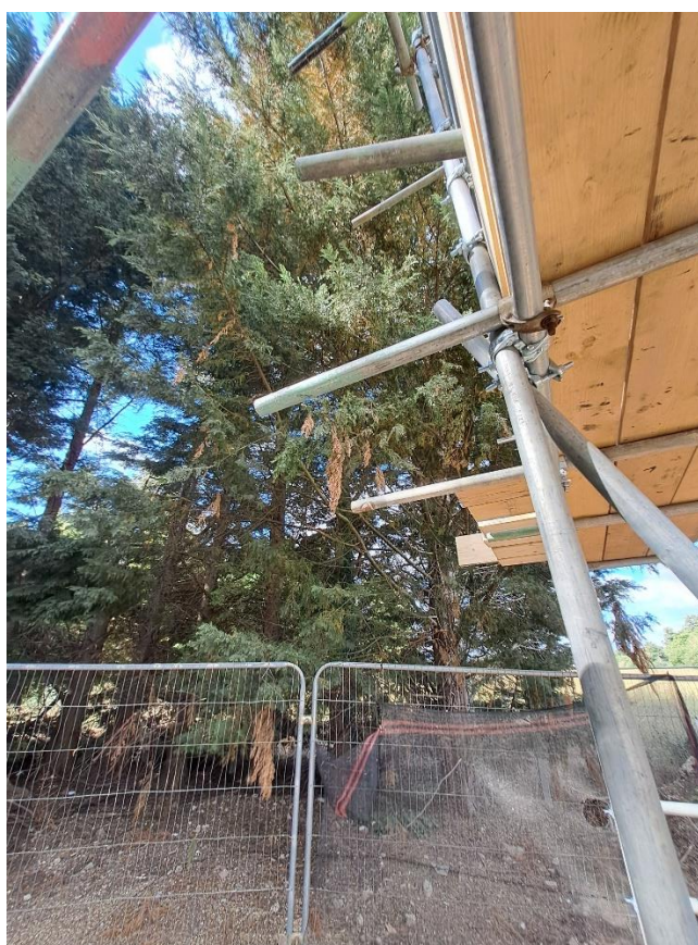
Photo 2 of G10 looking south-west
