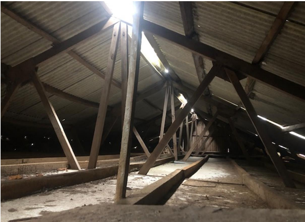
Internal roof truss profile.
