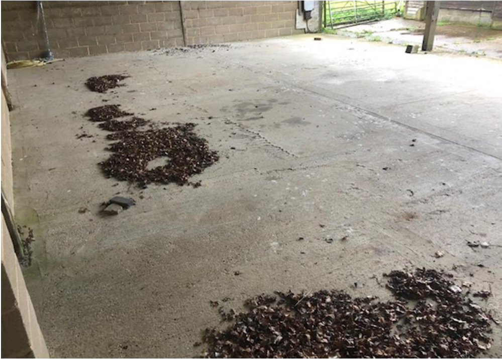
Ground floor slab to main barn.
