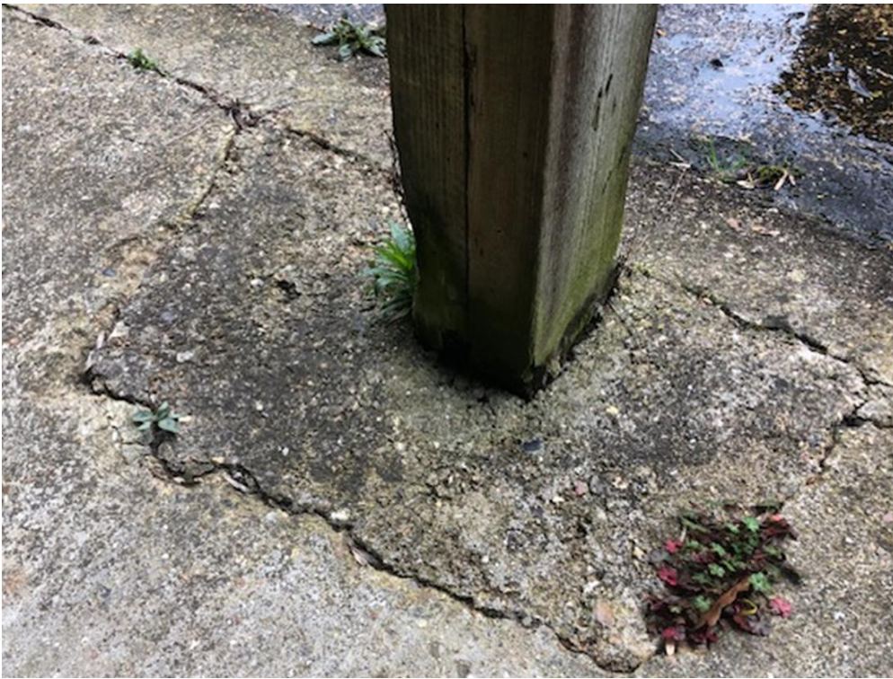
Timber post at ground level.
