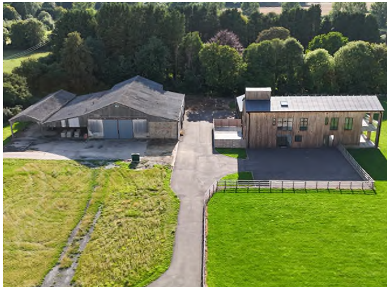
Image 6: View facing west towards the Cart Lodge. The Cart Lodge is screened from views. Landscape boundary provides further screening to the west.
