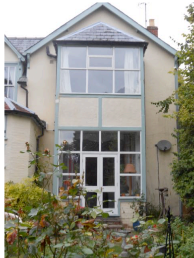
Existing 2 Storey Rear Extension
