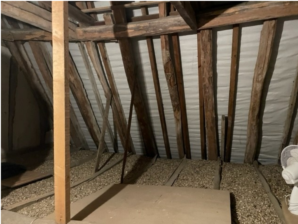
Before works undertaken - existing loft space with supports to the bowed/sagging ceiling joists and strut supporting the water tank platform above.
