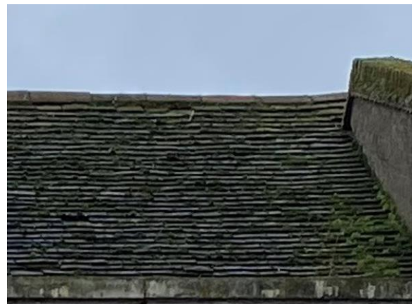
Front façade pitched roof tiles to be replaced like for like
