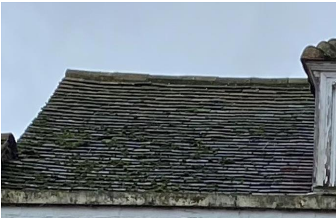
Front façade pitched roof tiles to be replaced like for like
