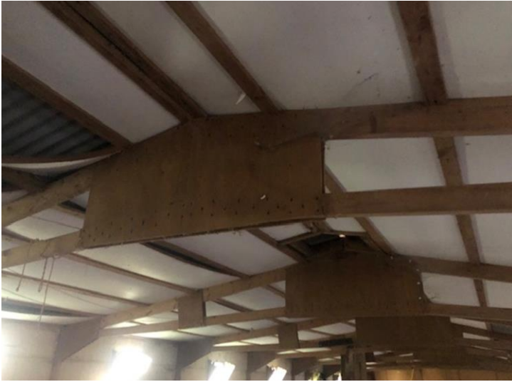
Main frame detail at ridge.
