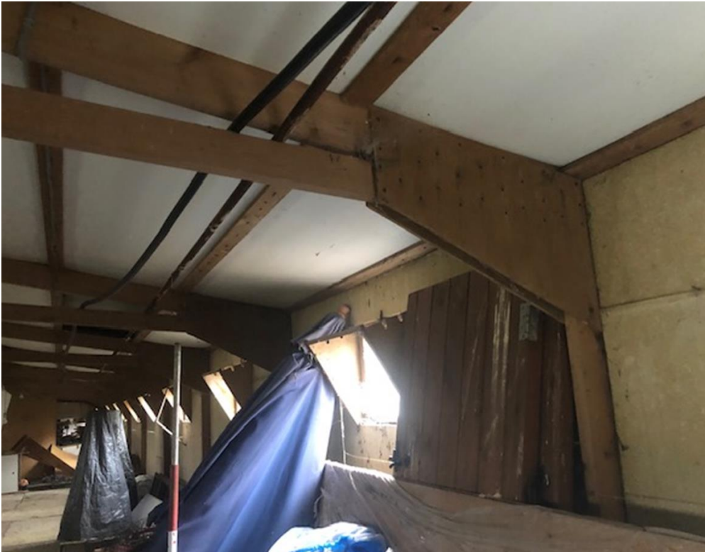
Main frame detail at eaves.
