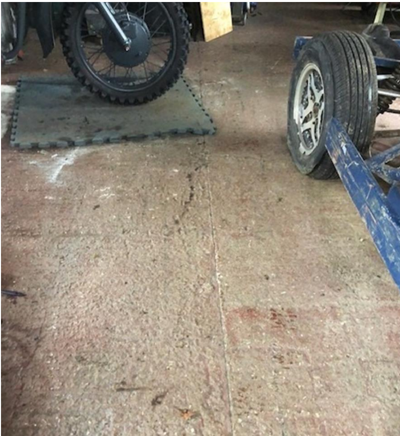
Concrete floor slab.
