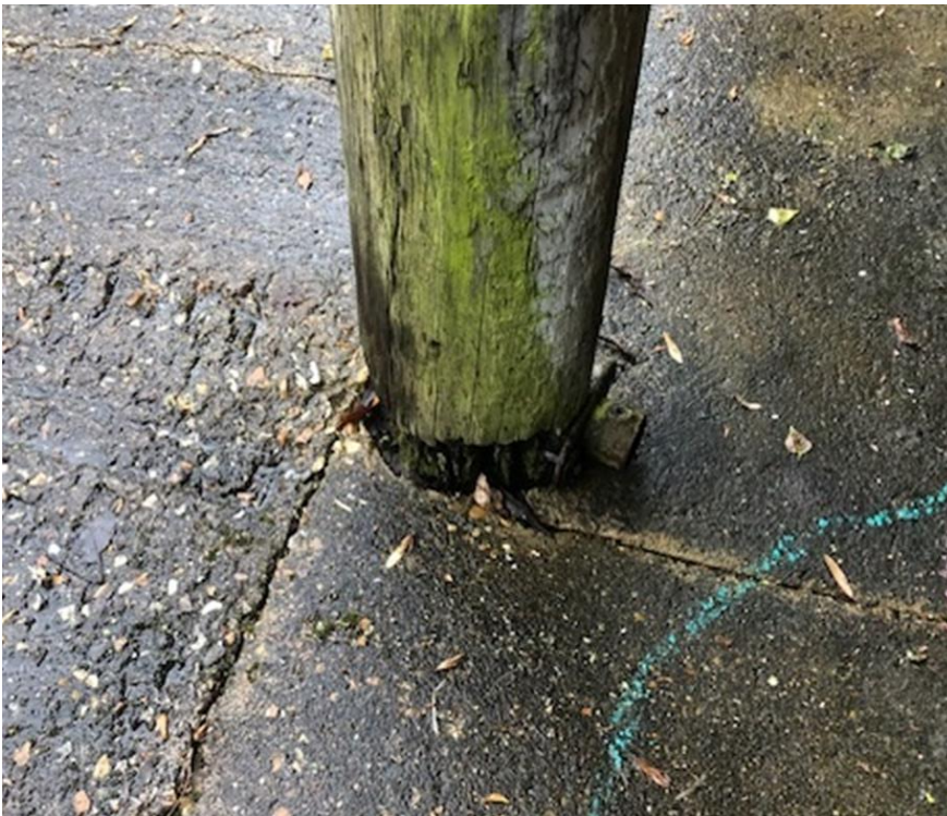
Timber post at ground level to lean to barn.
