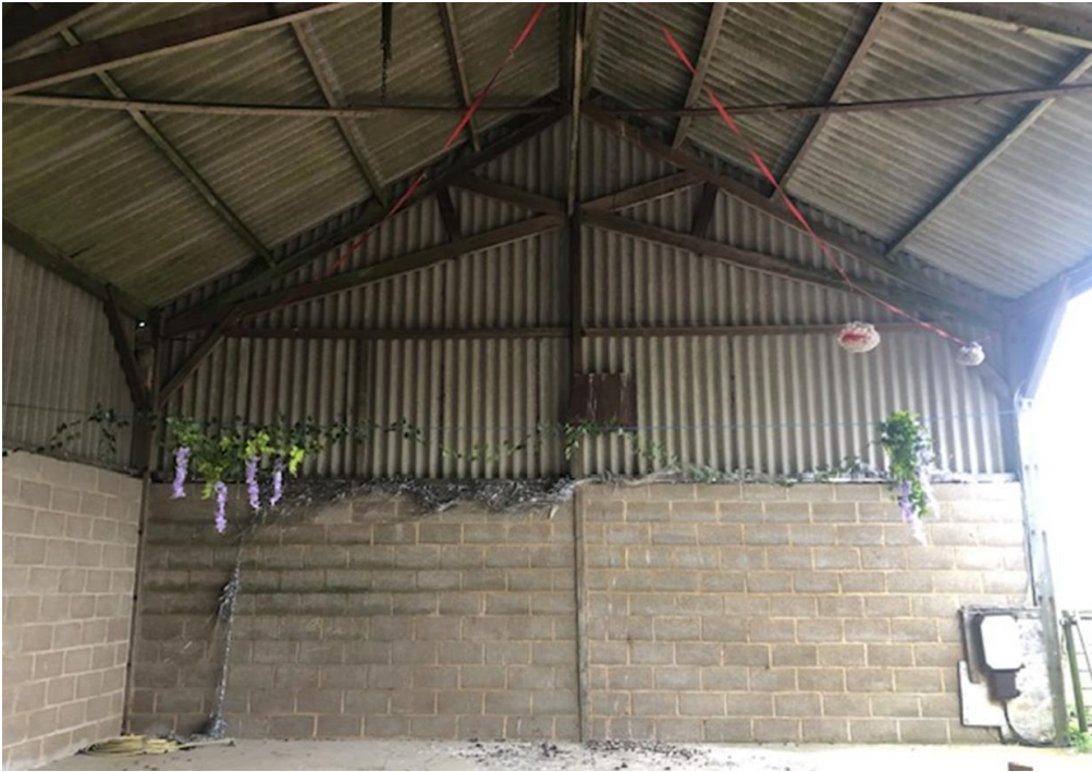
Internal framing to main barn.
