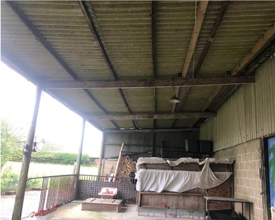
Internal framing to lean to barn.
