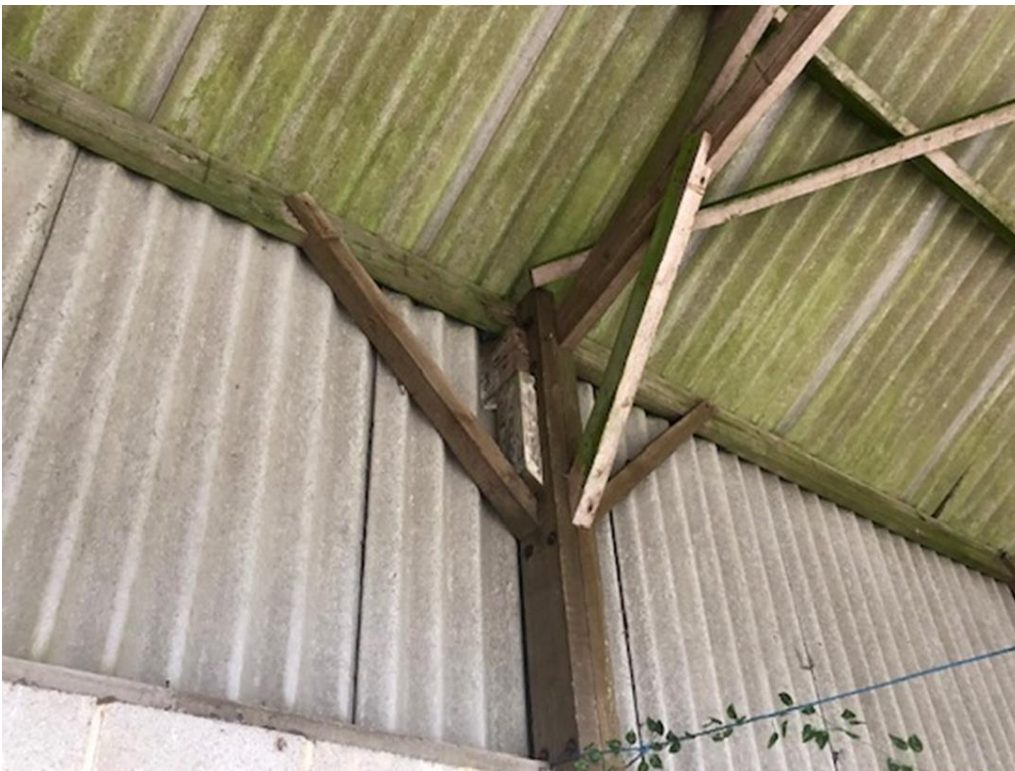
Roof truss arrangement at post.
