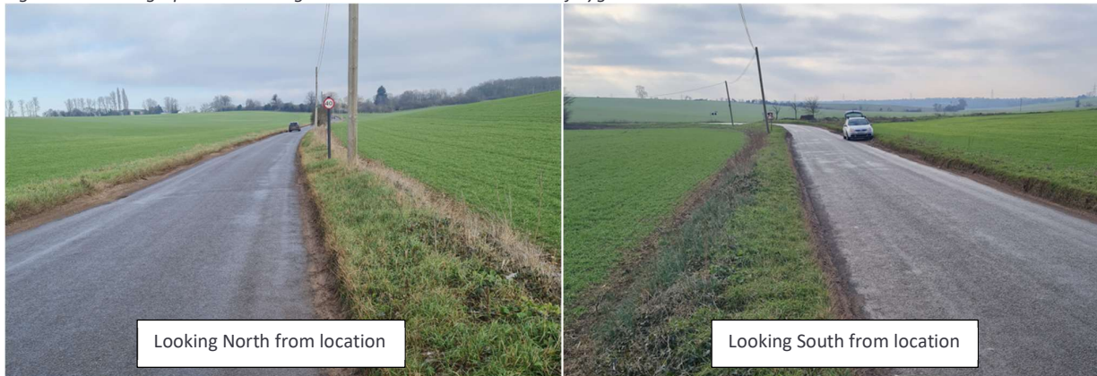
Figure 3-6: Photographs taken along narrower section to the south of Bygrave
