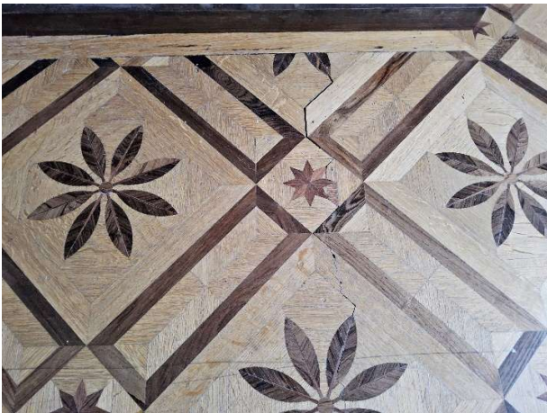
Separation of Joints and Cracking
