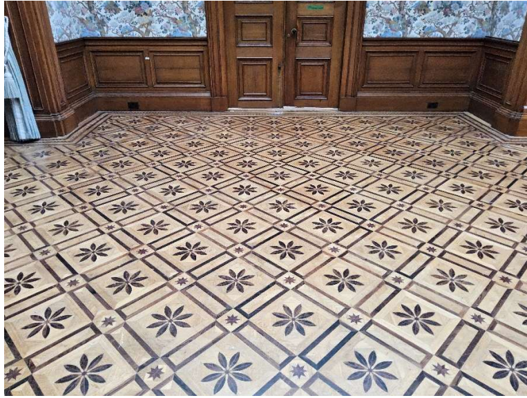
Existing Hall Floor
