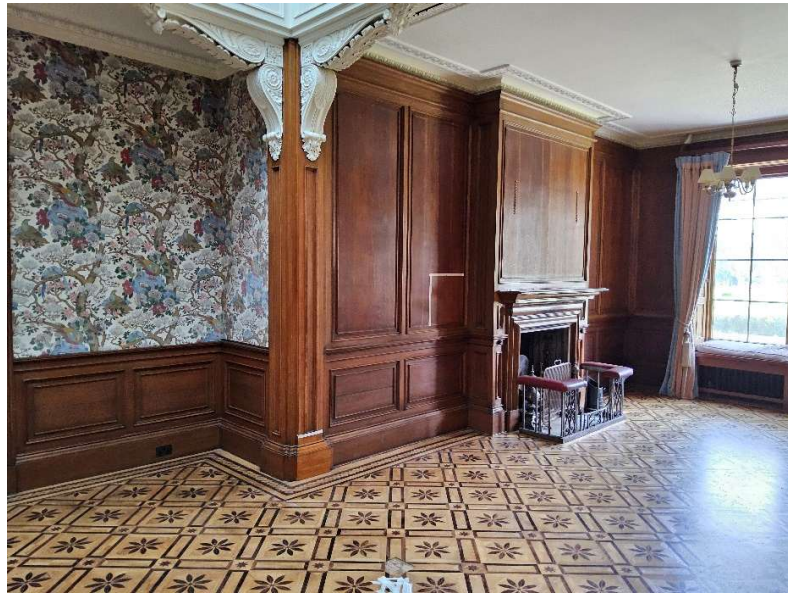
Timber Paneling to Hall
