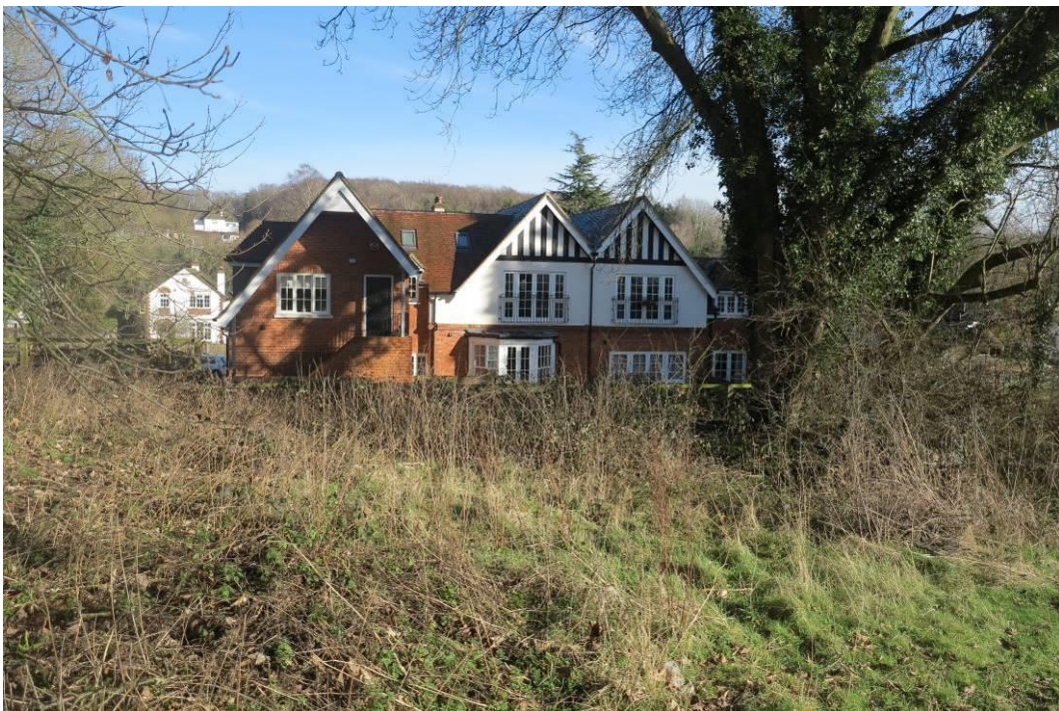
Plate 12. Existing buildings on the site
