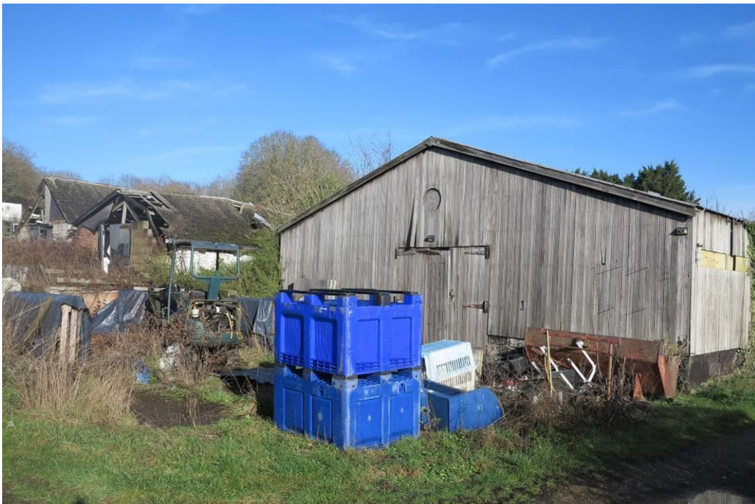
Plate 16. Existing buildings on the site
