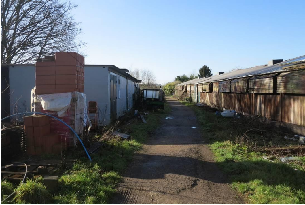
Plate 15. Existing buildings on the site
