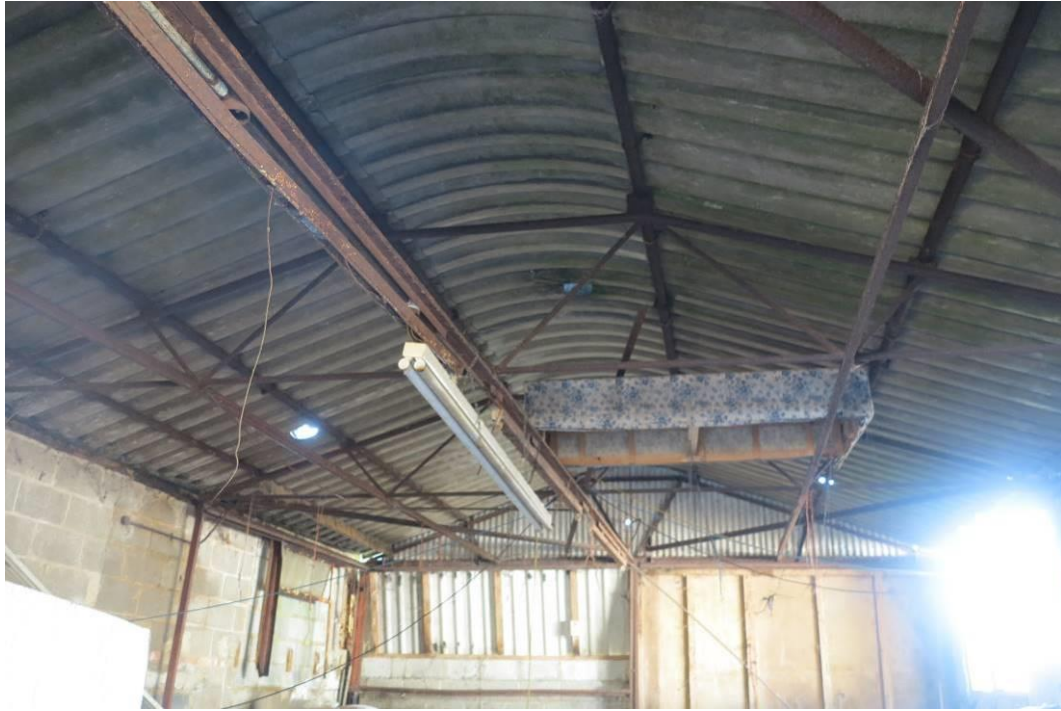
Plate 13. Existing buildings on the site
