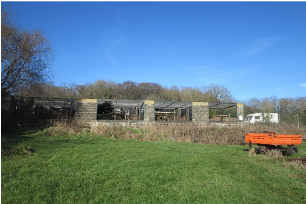
Plate 22. Existing buildings on the site
