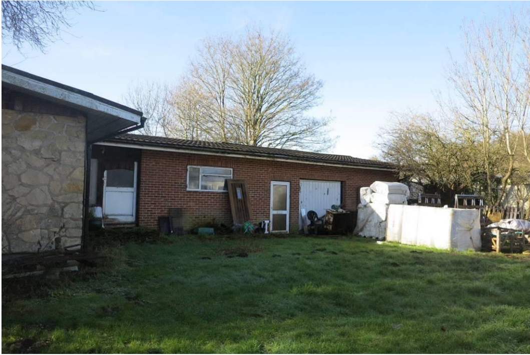
Plate 17. Existing buildings on the site
