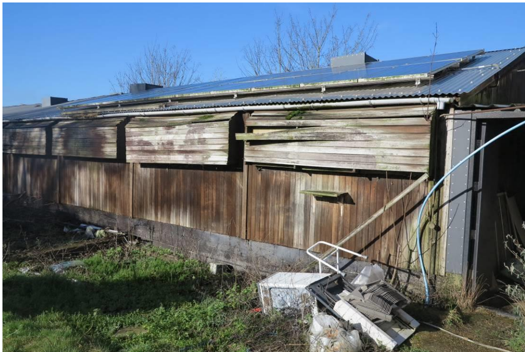
Plate 14. Existing buildings on the site
