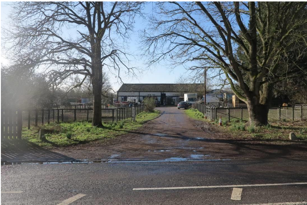
Plate 36. Looking towards the site from Codicote Road, with the main shed highly visible
