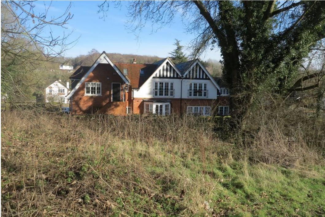
Plate 5. Looking towards the rear of 54 Codicote Road from the raised ground at the northern end of the site
