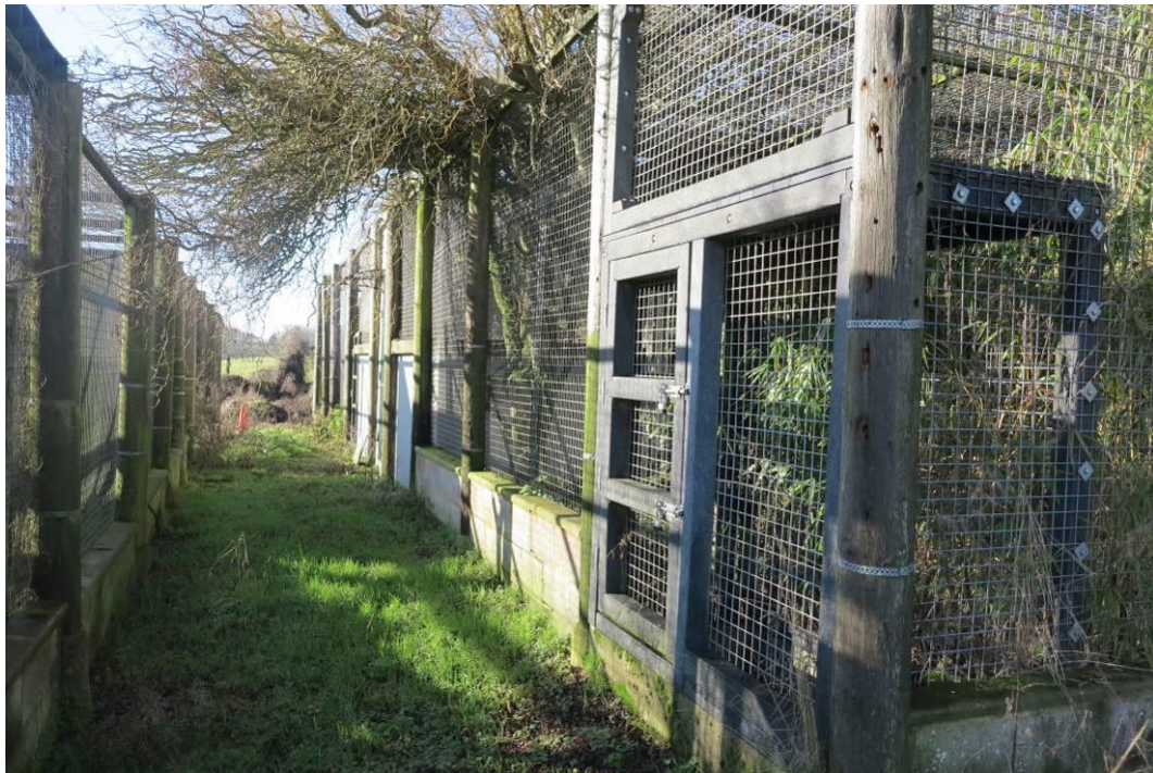
Plate 23. Existing buildings on the site
