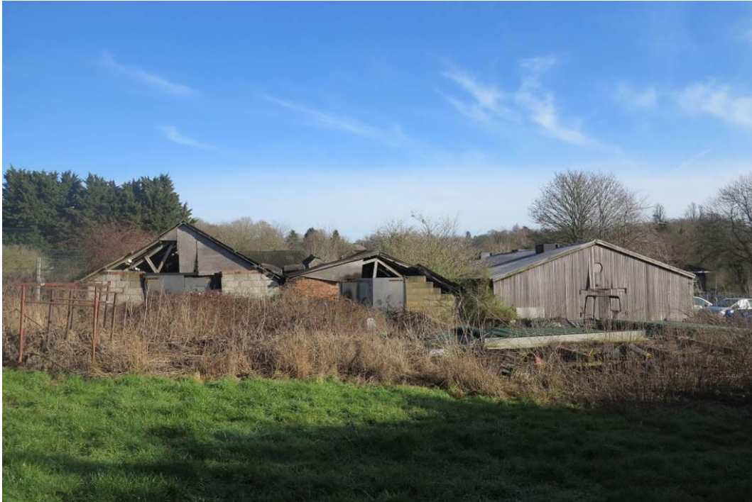
Plate 21. Existing buildings on the site
