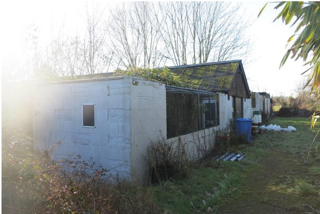
Plate 19. Existing buildings on the site
