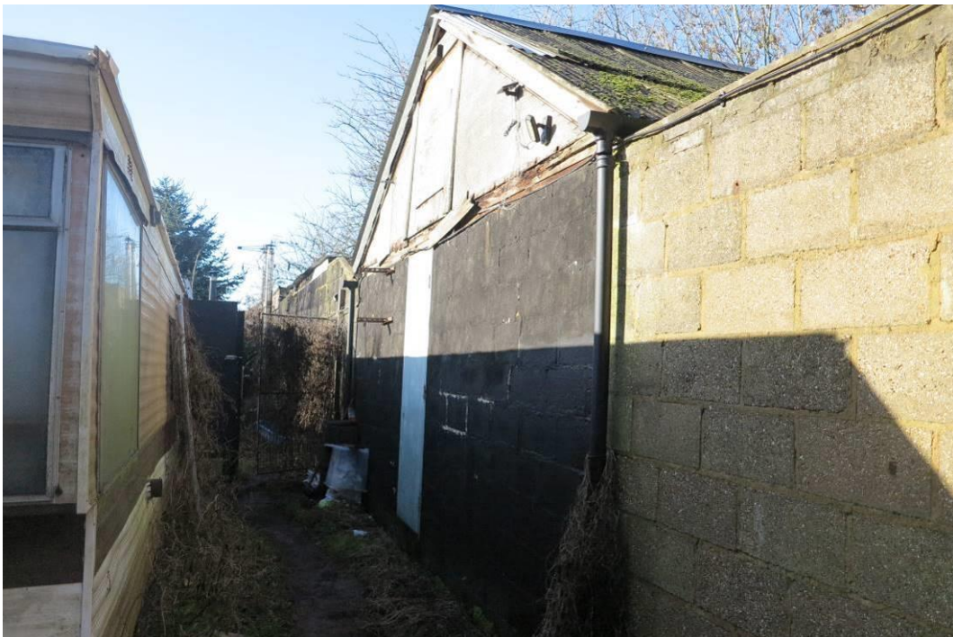
Plate 18. Existing buildings on the site
