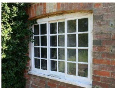
Detail of the replica horizontal sliding sash window and brickwork.
