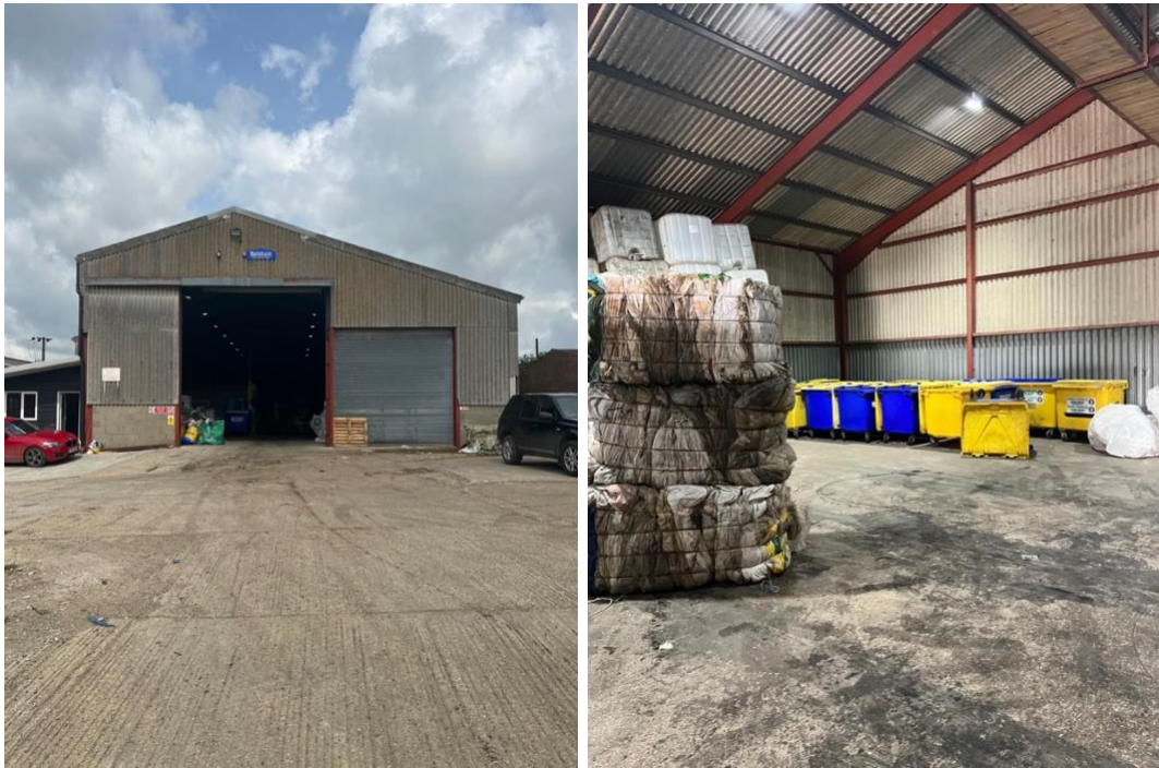
Figure 3-5 Exterior & Interior of B1
