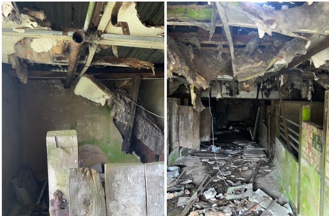
Figure 4-1 Interior of B2
