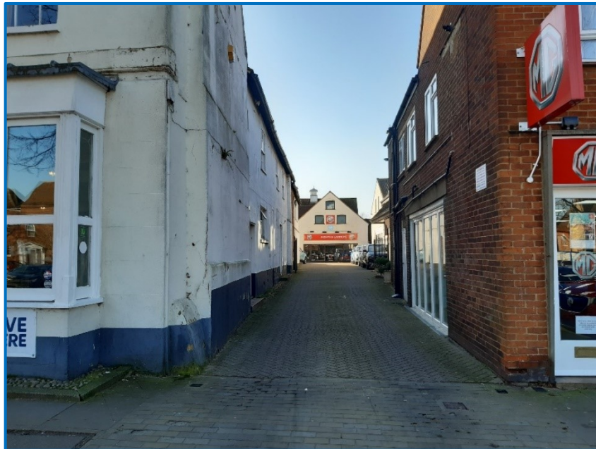
Figure 4 – Side access between the site and Brown & Gammons
