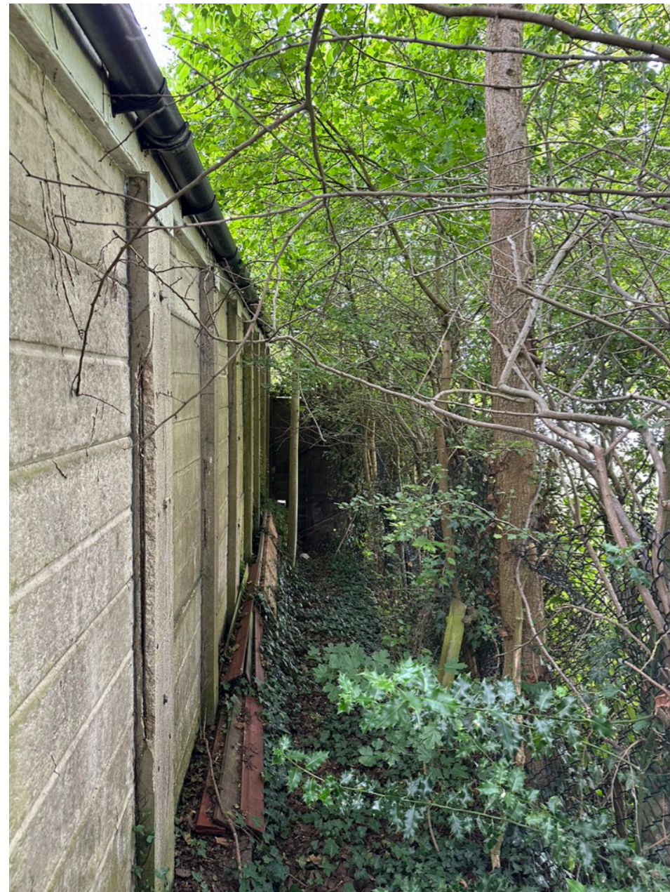
East facing external wall showing rainwater run off and trees and hedges on border
