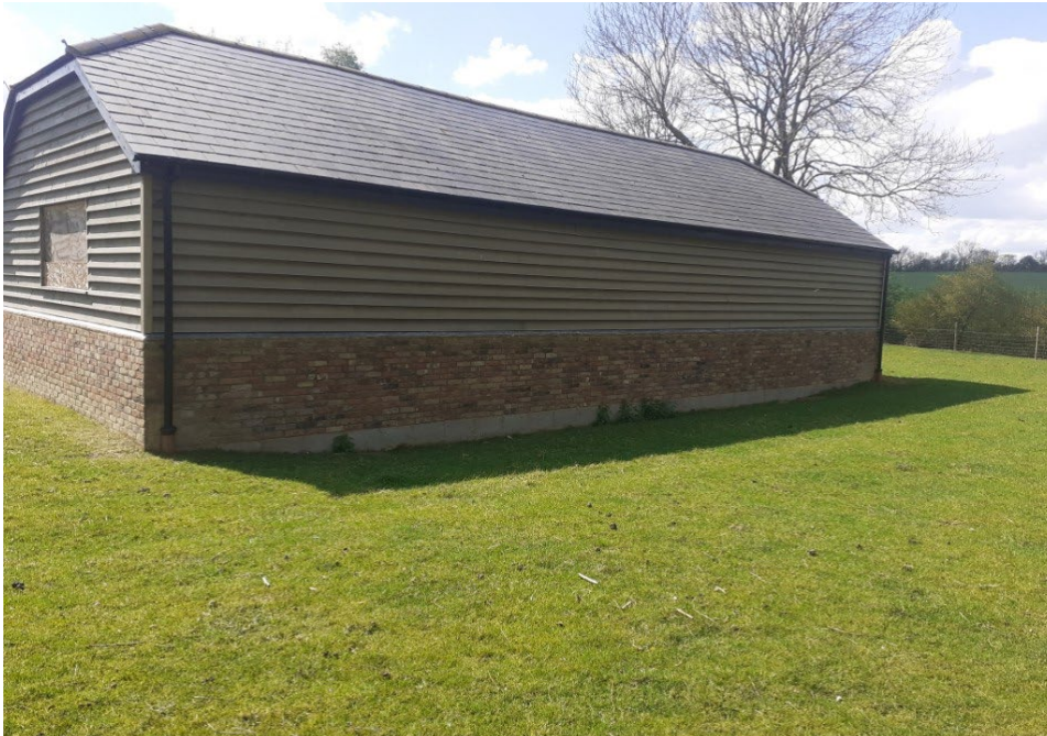
Photograph 3: View of the rear of the barn, facing south / southwest.
