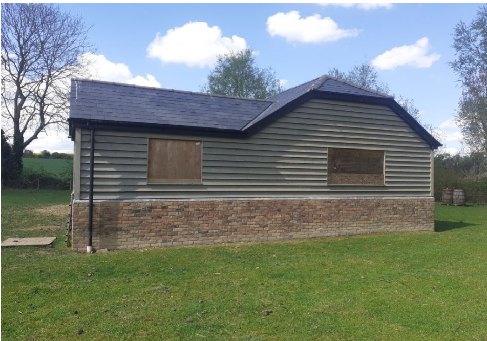
Photograph 4: View of the barn facing northwest.
