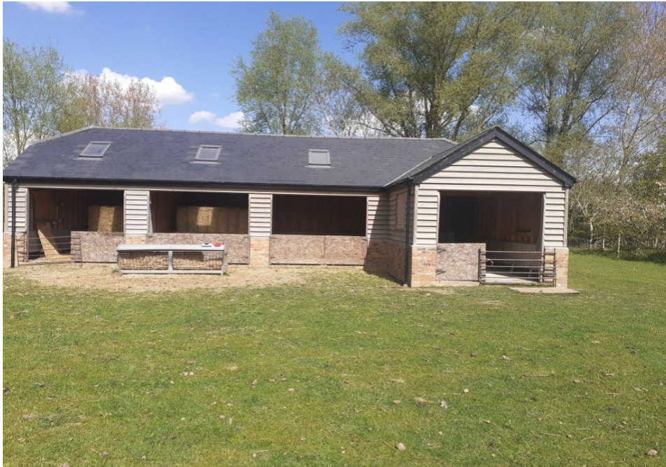
Photograph 1: View of the existing barn used for the housing of livestock, facing northeast.
