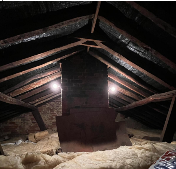
The existing chimney from within the loft
