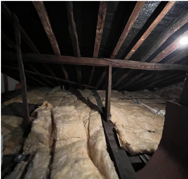
The existing roof structure from within the loft
