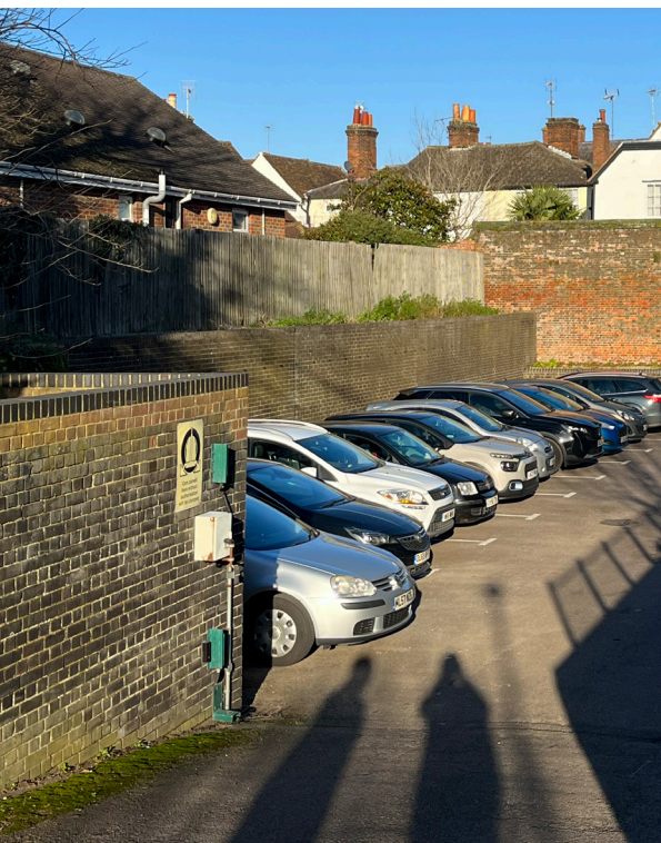
The rear elevation from Wratten Road East
