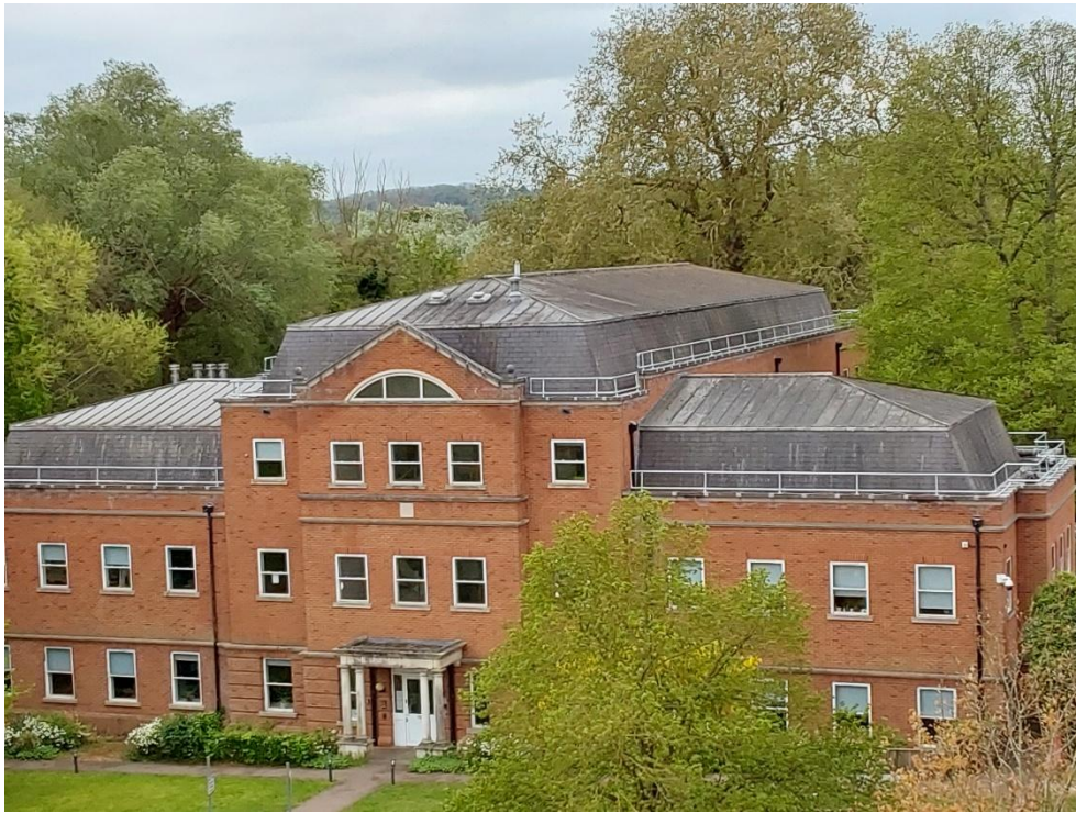
Photograph 1: Pease House (north-east aspect)
