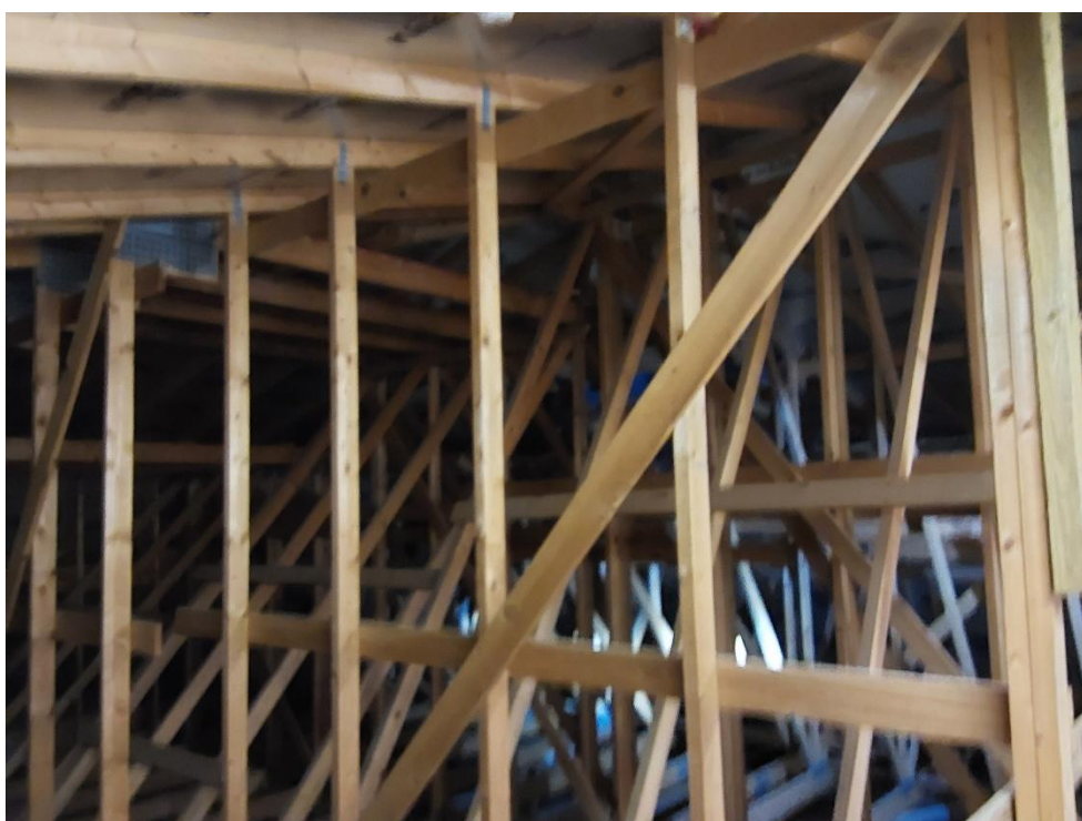
Photograph 6: Internal view of a roof cavity
