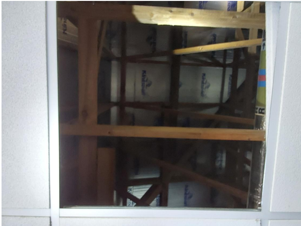
Photograph 7: Internal view of the main central roof cavity
