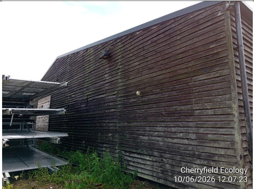
Figure 4: Rear of B1.
