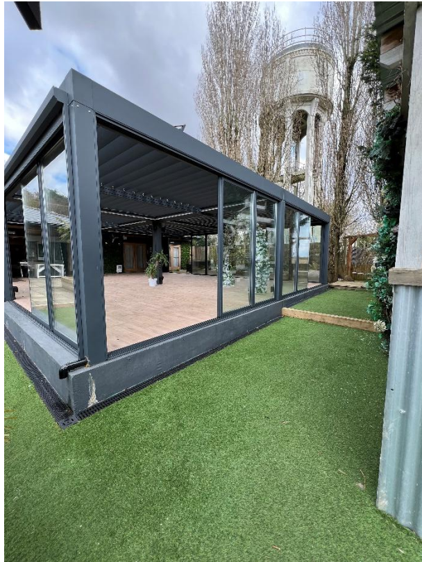
Rear elevation showing new louvre pod.
