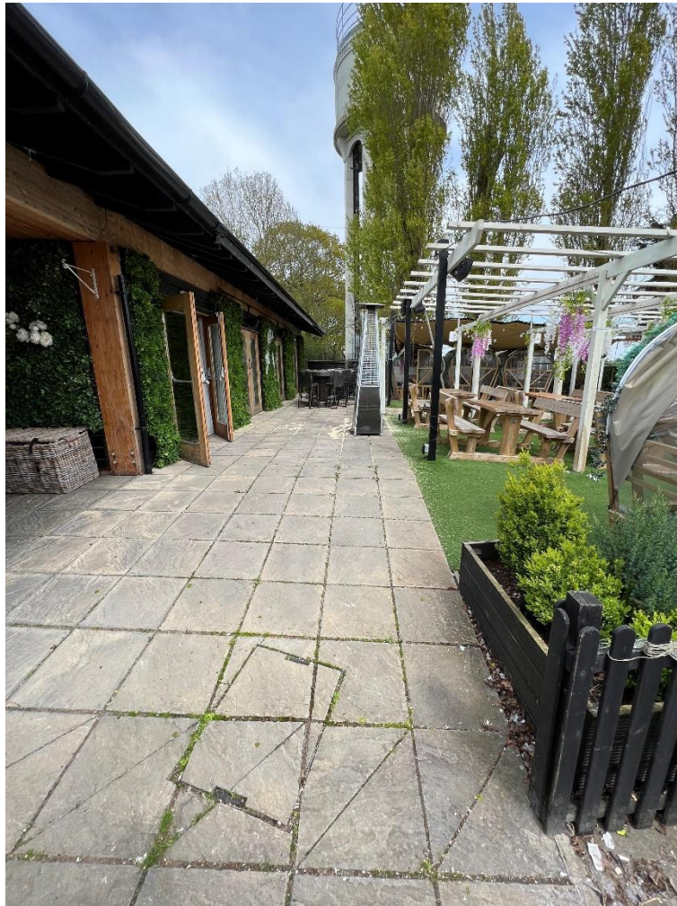
Existing rear elevation of function hall.
