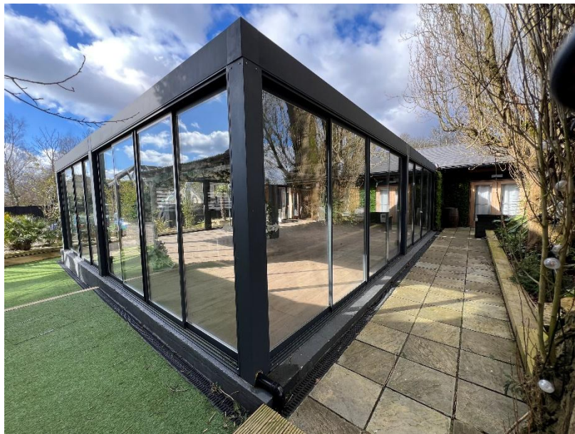
Rear elevation showing new louvre pod.
