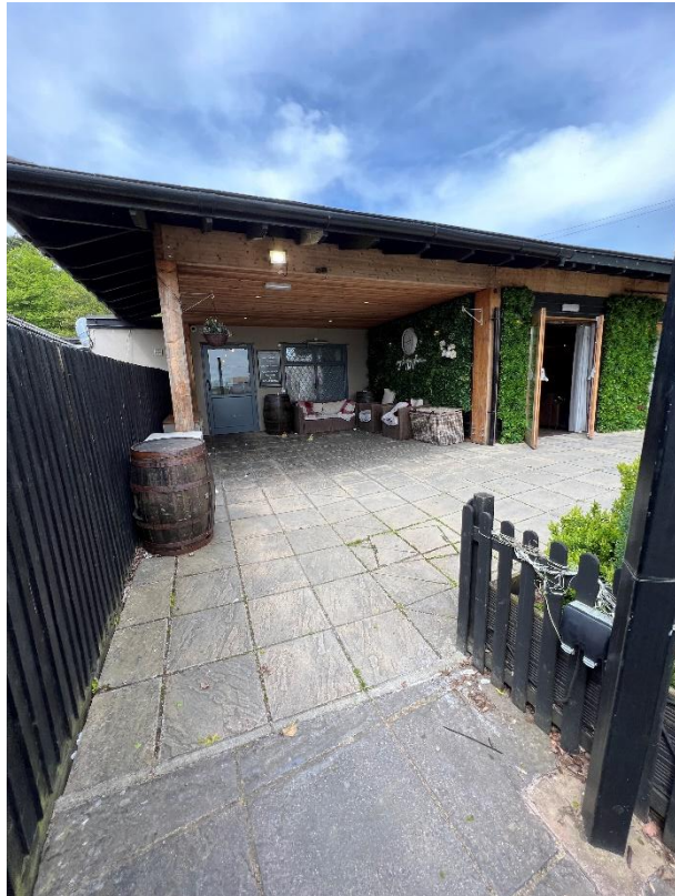
Existing rear entrance into Public House.
