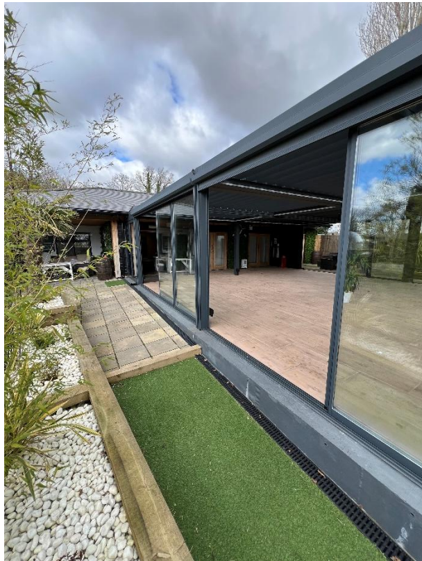
Rear elevation showing new louvre pod.
