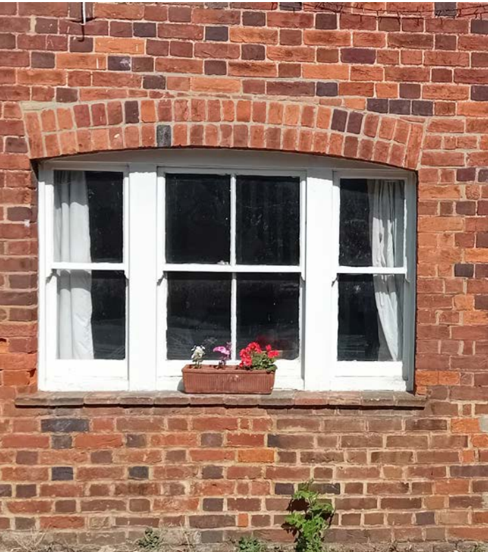
Multi-tone brickwork, brick arch headers
