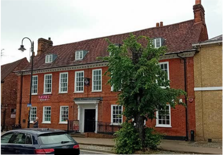
Lead dormers, cornice mouldings to eaves
