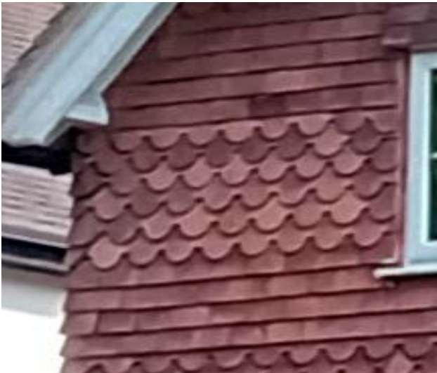
Tile Hanging with feature Club Tiles
