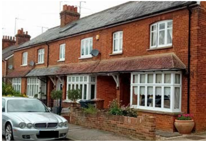
Hipped roof bay windows
