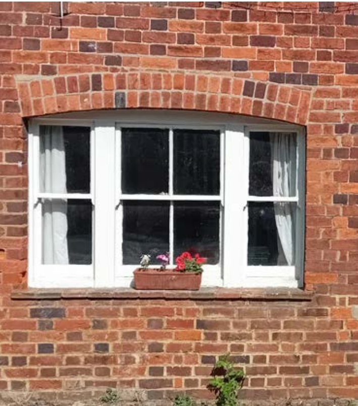
Multi-tone brickwork, brick arch headers
