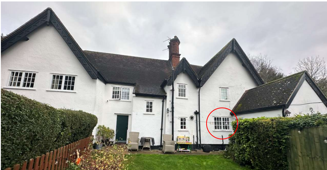
Photograph of existing rear elevation of 3 Letchworth Lane (window circled in red proposed for replacement)
