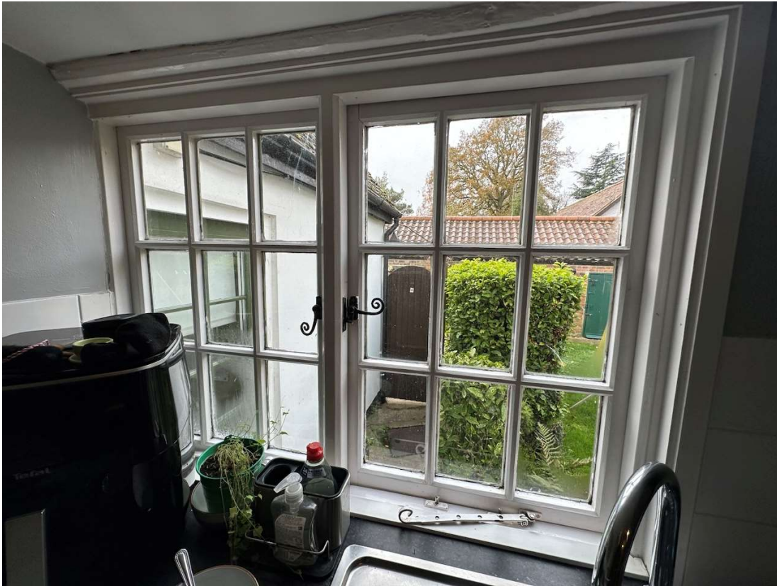
Internal photograph of ground floor rear window proposed for replacement
