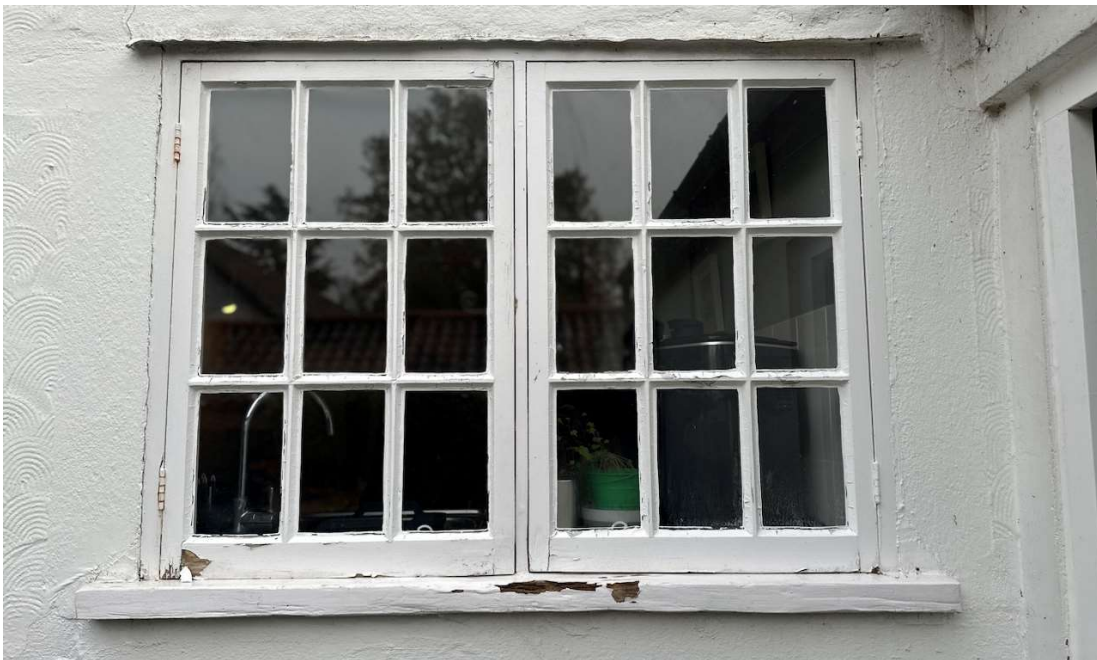
External photograph of ground floor rear window proposed for replacement
