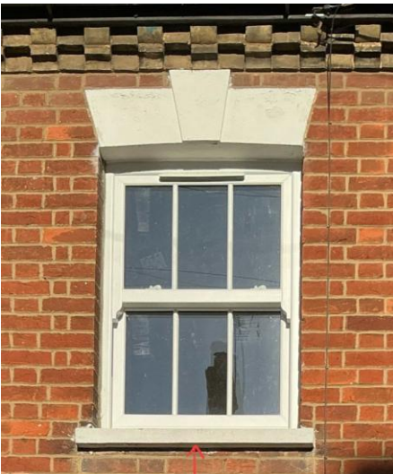
New window fitted at 19 Benslow Lane, that have been applied for and refused
