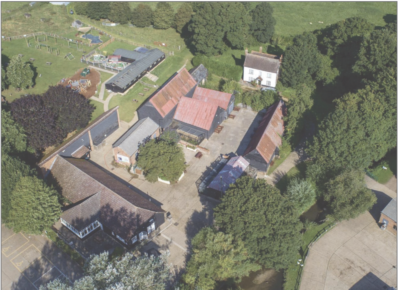
Standalone Farm: aerial view of farm buildings
