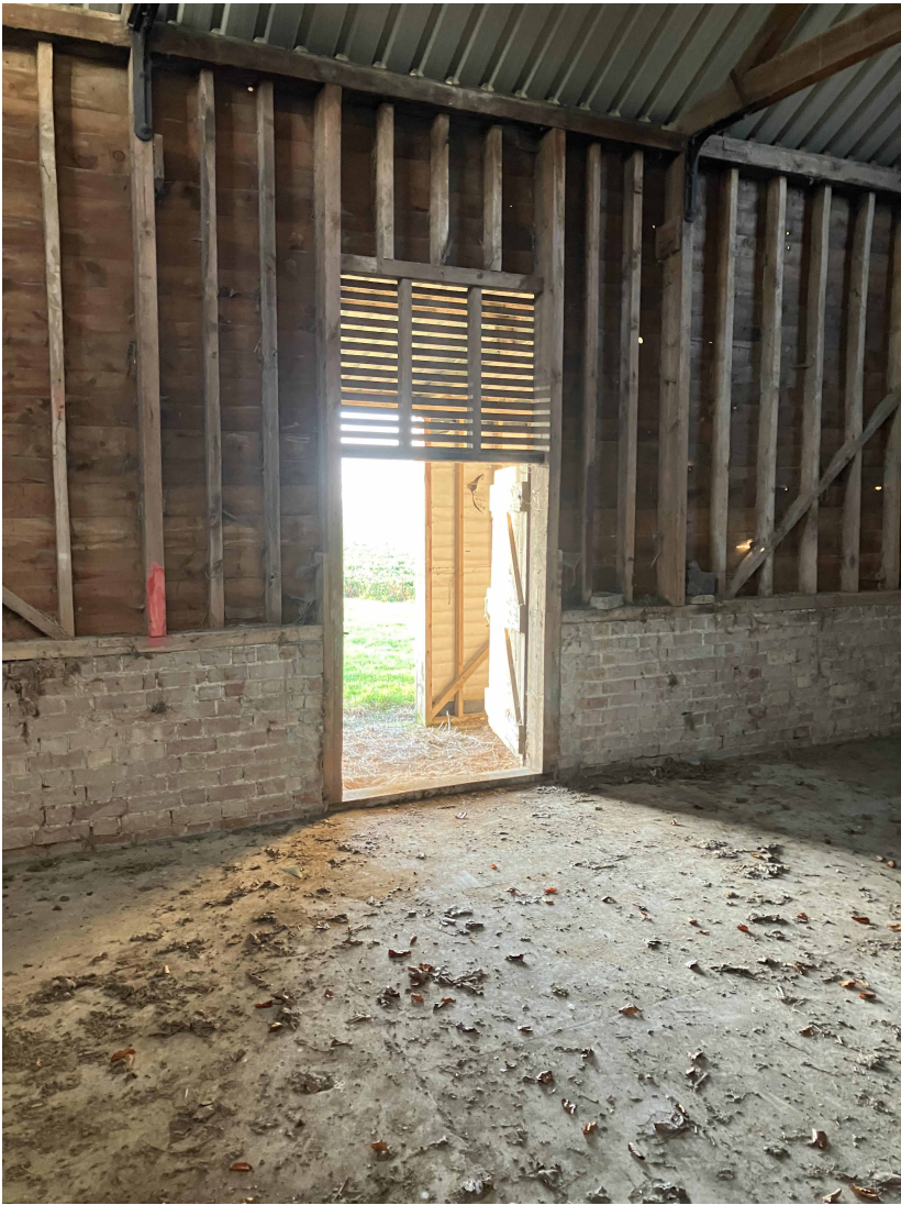
Internal feature wall
