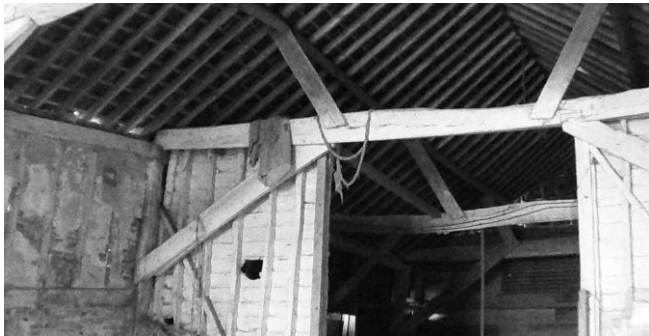
V3 B1b-4 surveyor photo
