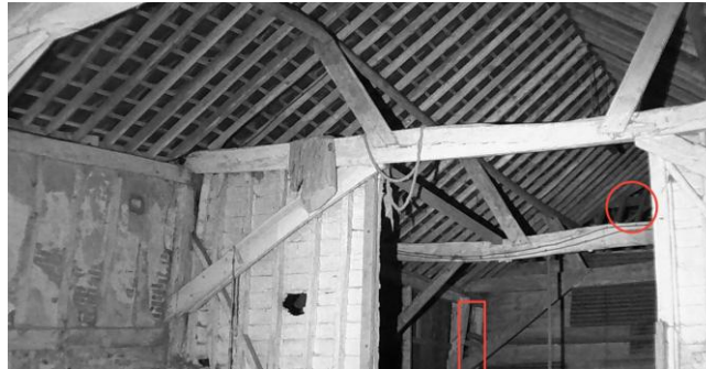
Roost 1& 2 – Internal entry and exit points
