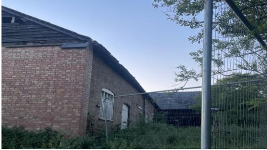
V2 B1b-1 surveyor photo
