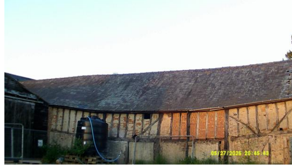
V2 B1b-3 surveyor photo
