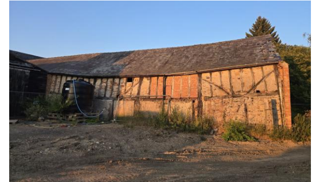
V3 B1b-3 surveyor photo
