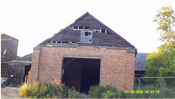
V3 B1b-2 surveyor photo
