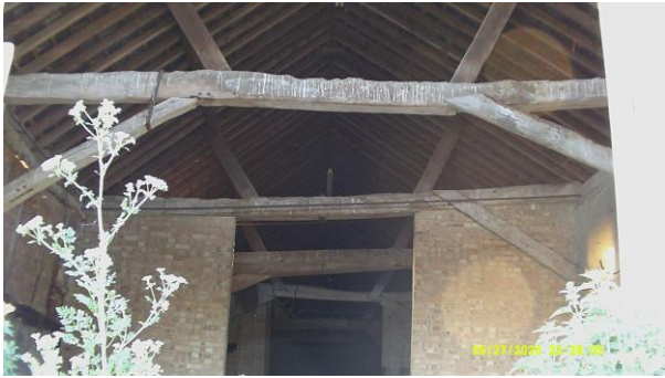
V2 B1b-4 surveyor photo
