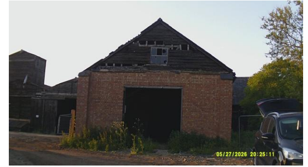
V2 B1b-2 surveyor photo
