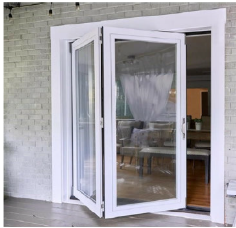
First Floor Bifold Doors
