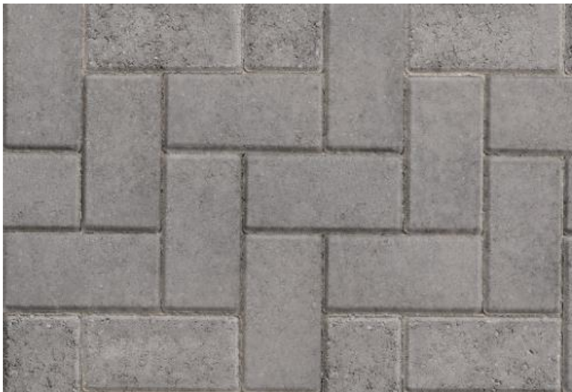
Marshall's Block Paving Colour – Natural (parking areas)
