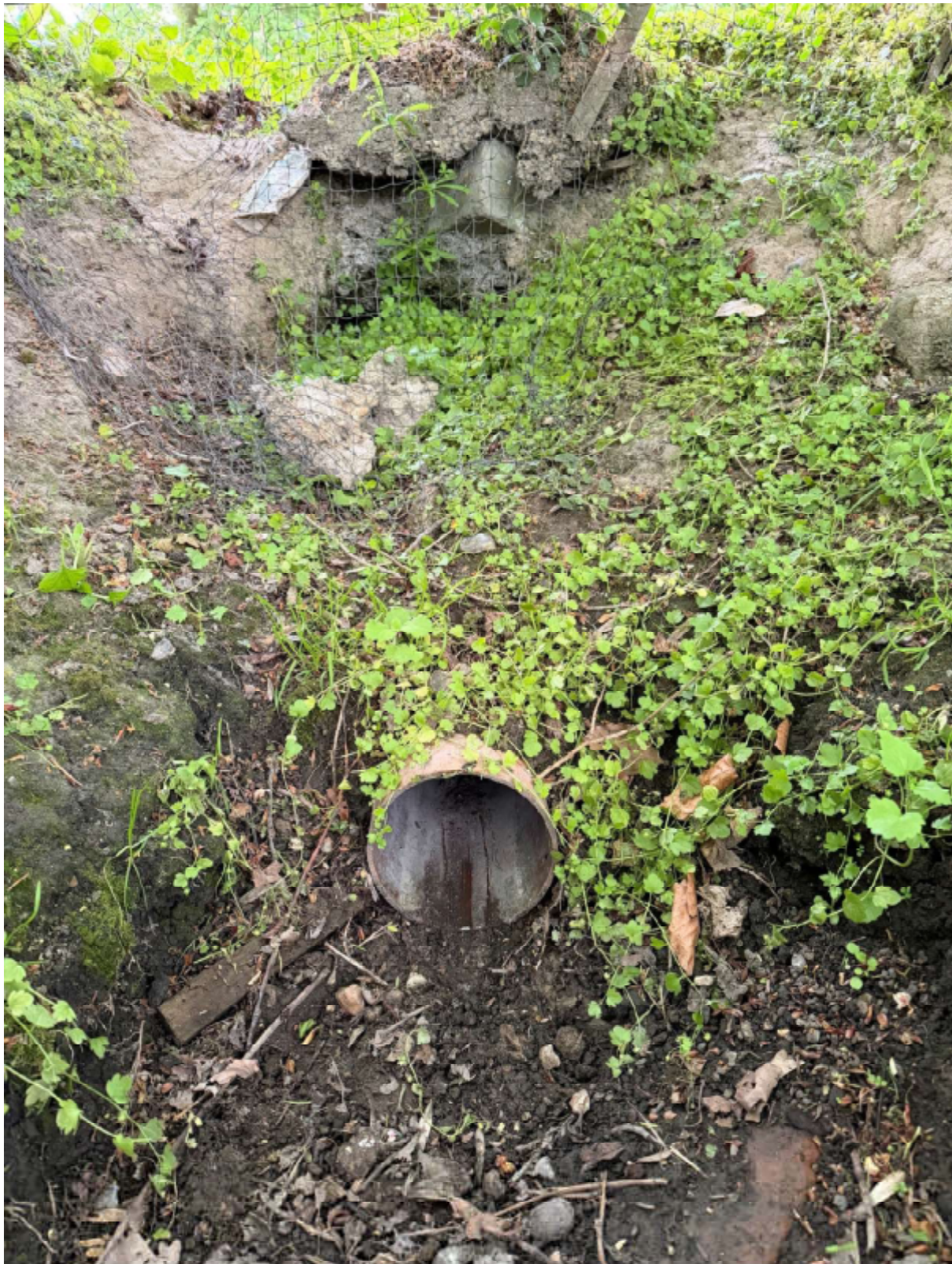
Photograph 2 – pipe entering application site (looking back towards Walnut Tree Road)
