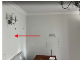
3.2.2 - Internal View from Lounge
