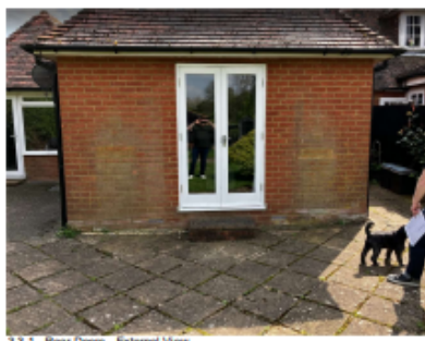
3.3.1 - Rear Doors - External View
