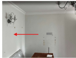
3.2.2 - Internal View from Lounge
