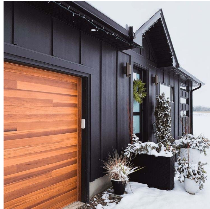
example of similar wall cladding & doors
