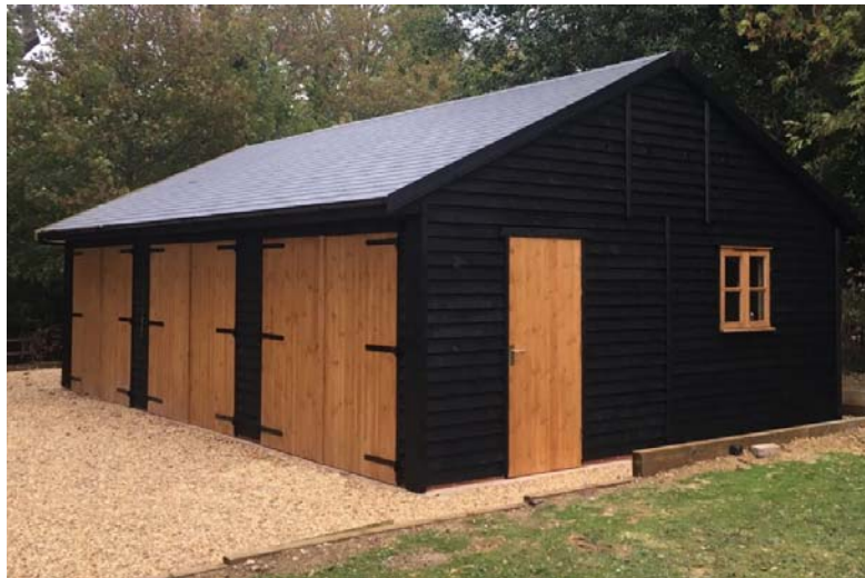
example of similar wall cladding & doors
