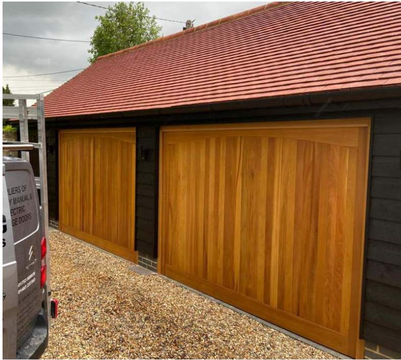
example of similar wall cladding, roof tiles & doors
