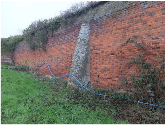
Fig.51 Brick buttresses and diaper brickwork
