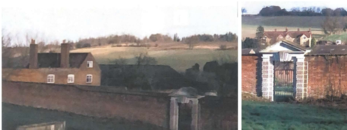
Figs.21-22 Boundary walls and entrances to Kitchen Garden LHS Hoo Farm RHS Entrance from former mansion site. [Source: Herts Gardens Trust]
