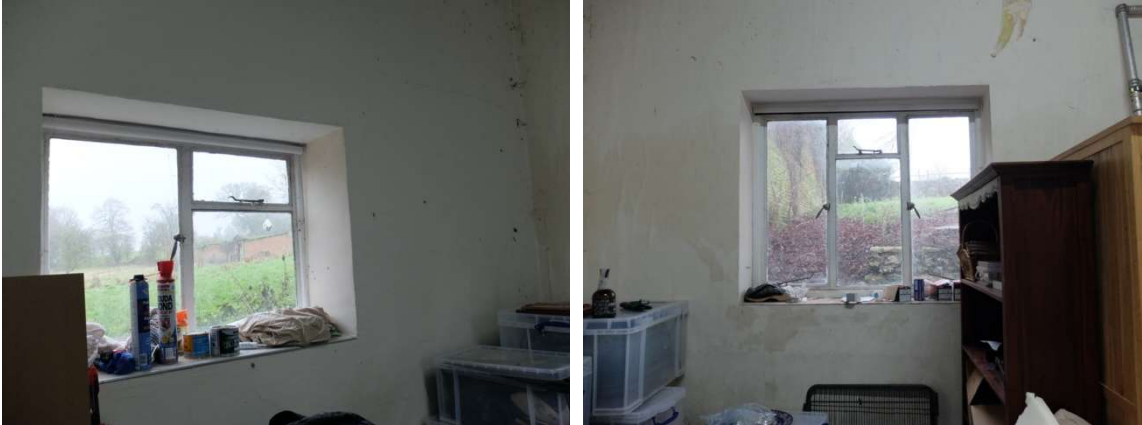
Fig.43 & 44 Metal-framed replacement windows in the former dairy.
