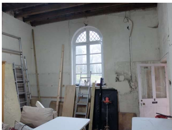
Fig.41 Arched window in the former dairy.
