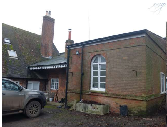
Fig.38 Former dairy with arched window
