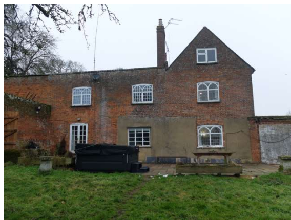
Fig.32 S facing with Gothic Revival feature windows
