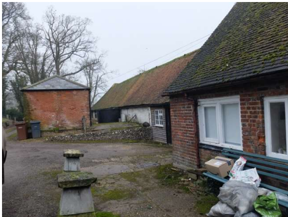
Fig.35 Looking N towards farm outbuildings
