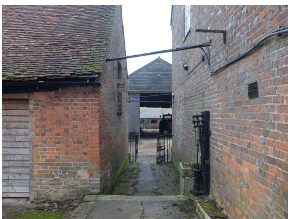
Fig.37 Change of level sloping from E to W
