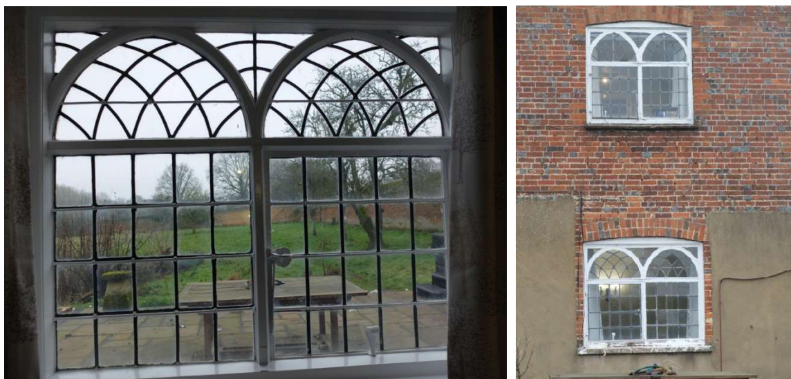
Fig.39 & 40 Gothic Revival influenced glazing on S elevation of farmhouse: timber frames and lead comes.
