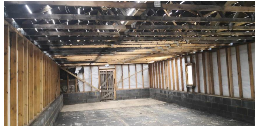
Figure 4. Interior of B1 , facing north. Exposed construction paper visible throughout. Breathable membrane visible at left of northern elevation.
